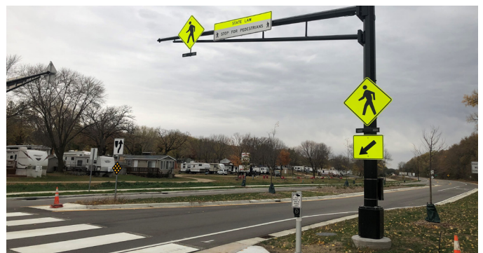
Highway 61 in Lake City, MN, showing a Rectangular Rapid Flashing Beacon and improved crosswalk
