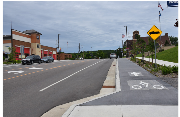
Hwy 28 (Minnesota Ave.) in downtown Glenwood, showing lane adjustment, raised cycletrack, and landscaping
