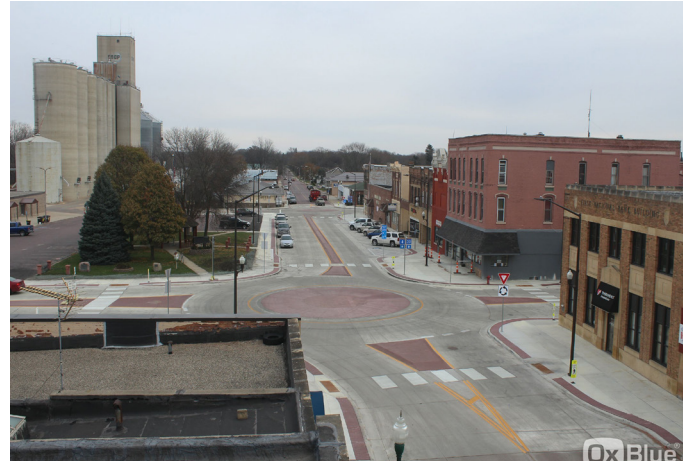
Highway 24 in St. James after construction, showing mini-roundabout, back-in angle parking and improved crosswalks
