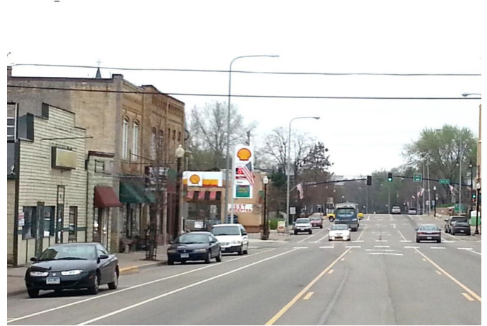
Highway 21 in downtown Jordan after construction, showing lane adjustment and bike lanes
