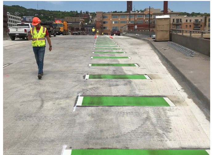
Lake Ave. bridge over Hwy 35 during construction, showing green-striped bike lane and new sidewalk
