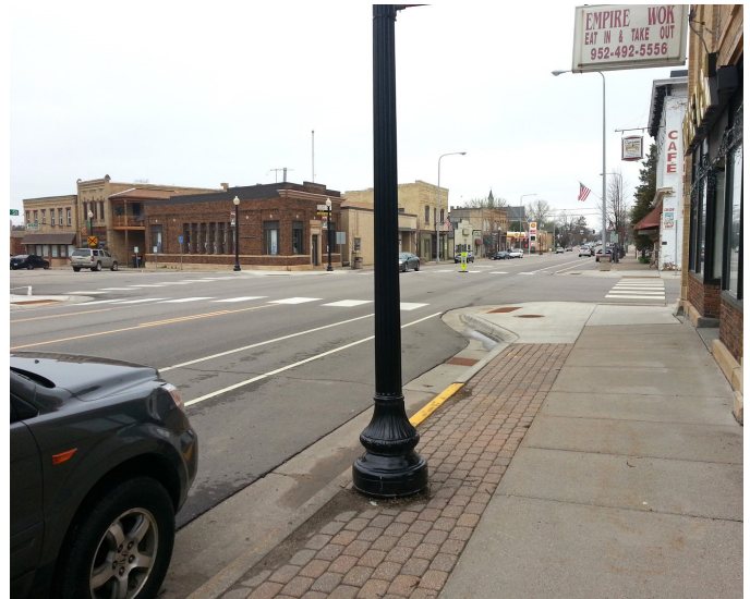
Intersection in downtown Jordan, showing bike lane, curb extension, and improved crosswalk
