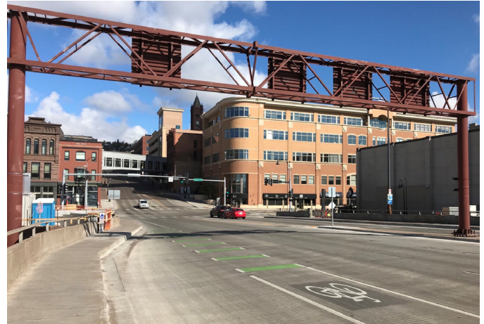
Lake Ave. bridge over Hwy 35 after construction, showing bike lanes, sidewalk, and lane adjustment
