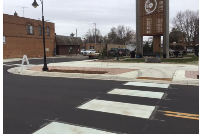
An intersection along Hwy 24 after construction, showing curb extensions, new sidewalk and decorative pavers, and improved crosswalks
