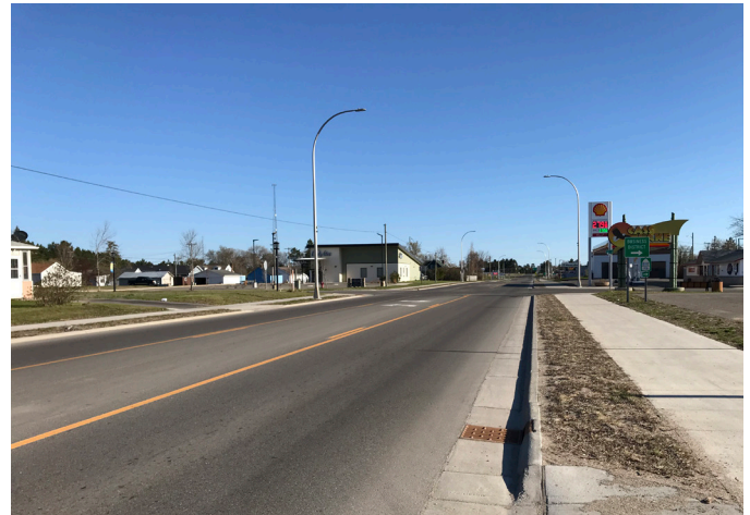
Highway 371 after construction, showing a new sidewalk (left), lane adjustment, and shared-use path (right).
