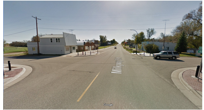
Highway 4 in Cosmos, MN after construction, showing curb extensions and lane adjustment
