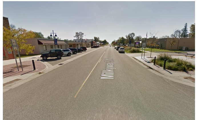
Highway 4 in Cosmos, MN, showing curb extensions, landscaping, and lane adjustment
