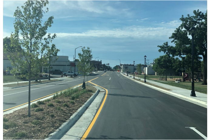
Highway 61 in Lake City, MN after construction, showing planted median, roadway reallocation, sidewalks, and shared-use path
