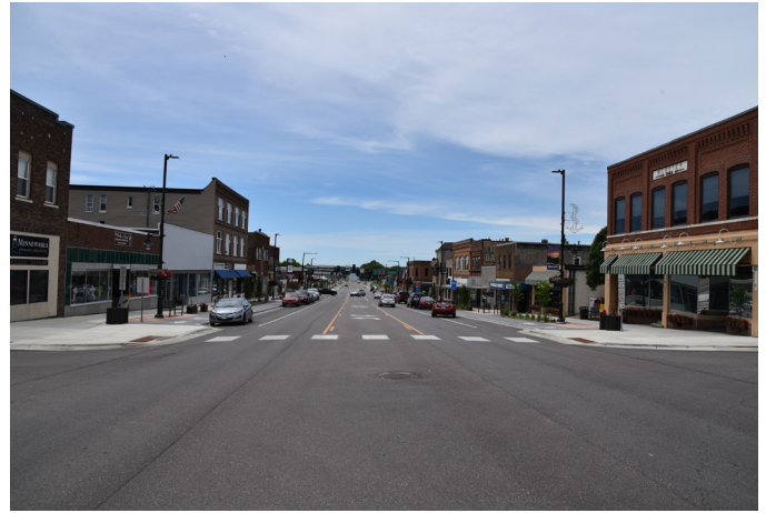
Hwy 28 (Minnesota Ave.) after construction, showing lane adjustment, raised cycletrack, bumpouts, and improved crosswalk
