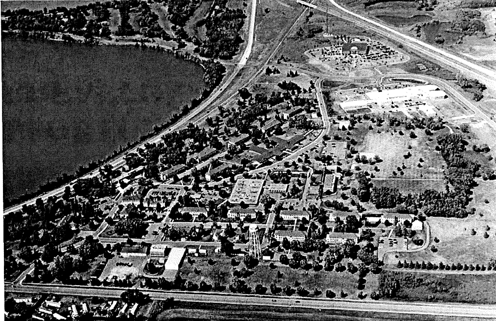
HISTORIC WILLMAR REGIONAL TREATMENT CENTER
