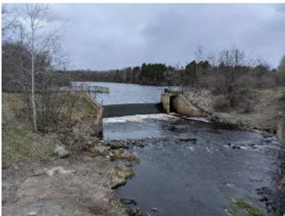
Photo 6. Grindstone Dam, viewing northwest
