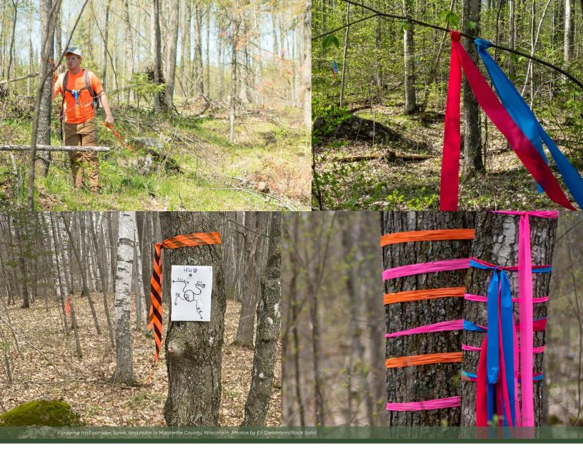
Flagging trail corridors is performed using a clinometer to confirm grades and ensure the corridor placements support the user objectives and trail types defined during the planning phase. While trail corridor flagging may seem simple, a professional trail planner must consider all of the information gathered up to this point and attempt to create a corridor that:
