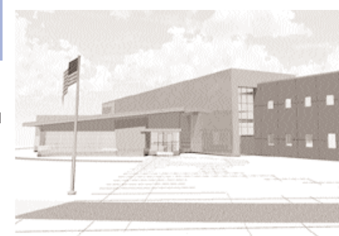
Minnesota's newest prison, the Minnesota Correctional Facility-Rush City, will open in January, 2000.
