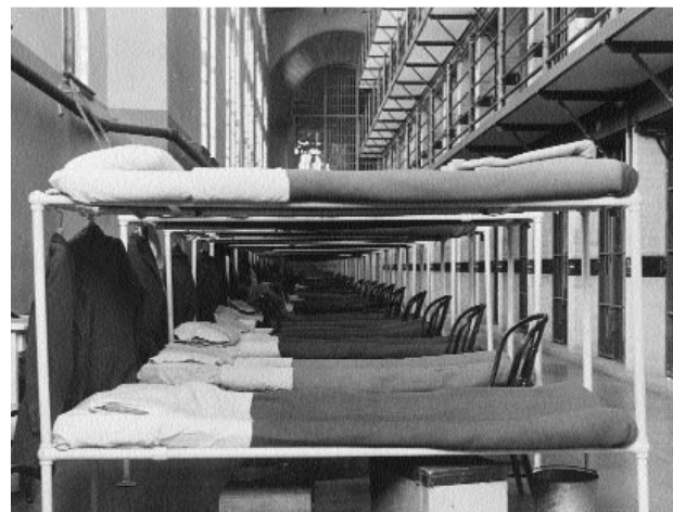
Cellhouse A at St. Cloud State Reformatory in 1923.
