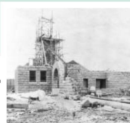
State Reformatory under construction in 1895.
