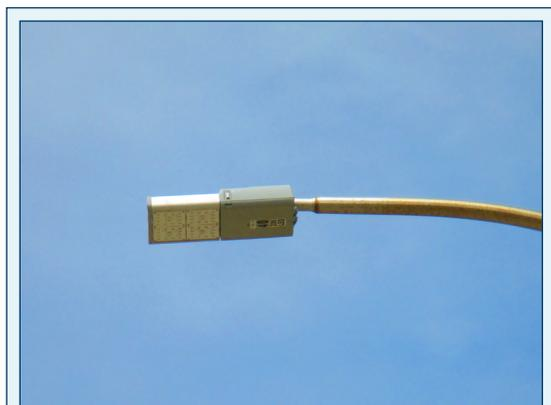
📷 LED luminaire installed on a light post on MnDOT right of way
