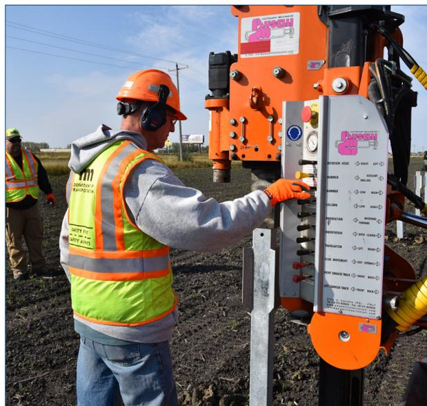
Ⓜ The Pauselli machine is a self-propelled pile driver used to install galvanized sleeves into the ground that support snow fence posts.
