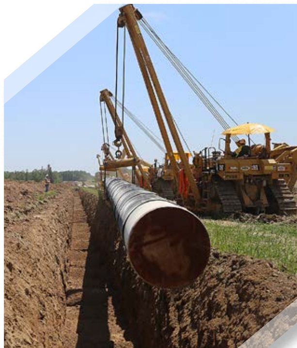
The Line 3 replacement project involved a large area of northern Minnesota.
