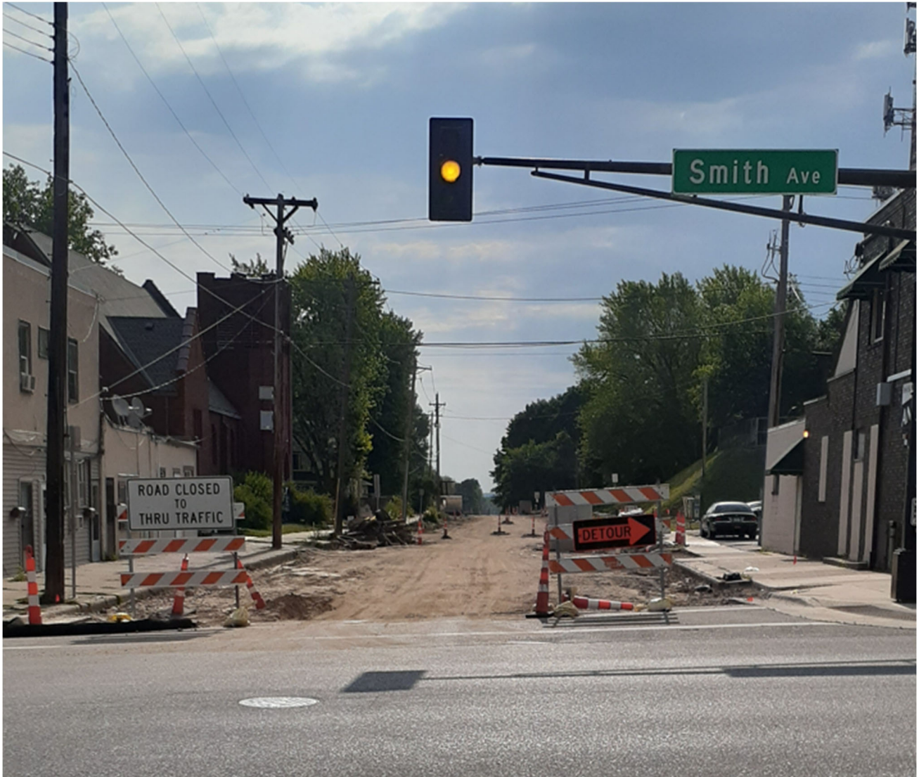
Annapolis Street Reconstruction: St. Paul / West St. Paul
