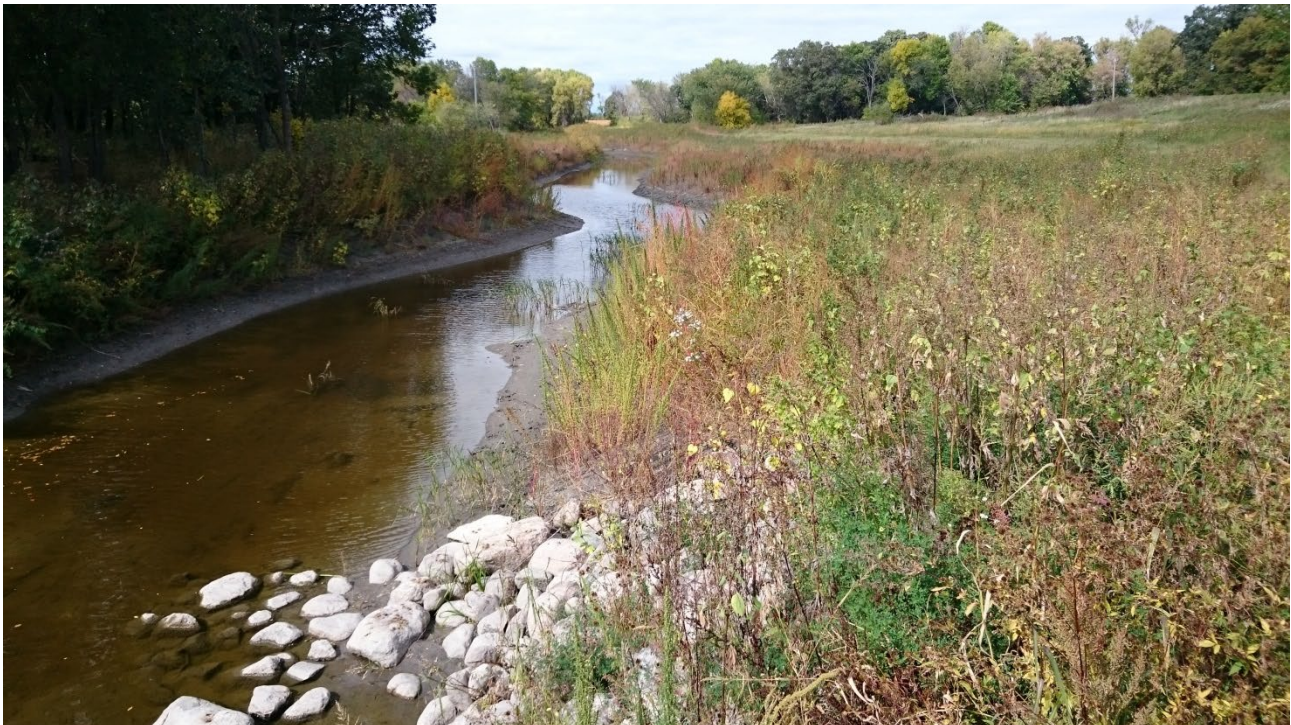
SR Photo 23: Riffle Boulder Vane below railroad car bridge.
