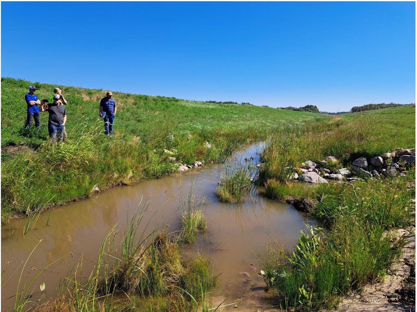
Photo 103. Looking east along 2-stage ditch where spring rains washed out 3 riffles at Bostic Creek (Bostic Creek Grade Stabilization, photo taken during site visit 8/30/2022).
