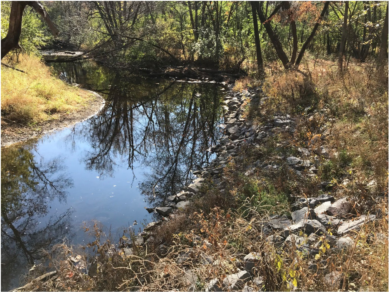
Figure 62. Stabilization Area 1 showing riprap toe and vegetated floodplain bench. Photo taken on 10/28/2022.
