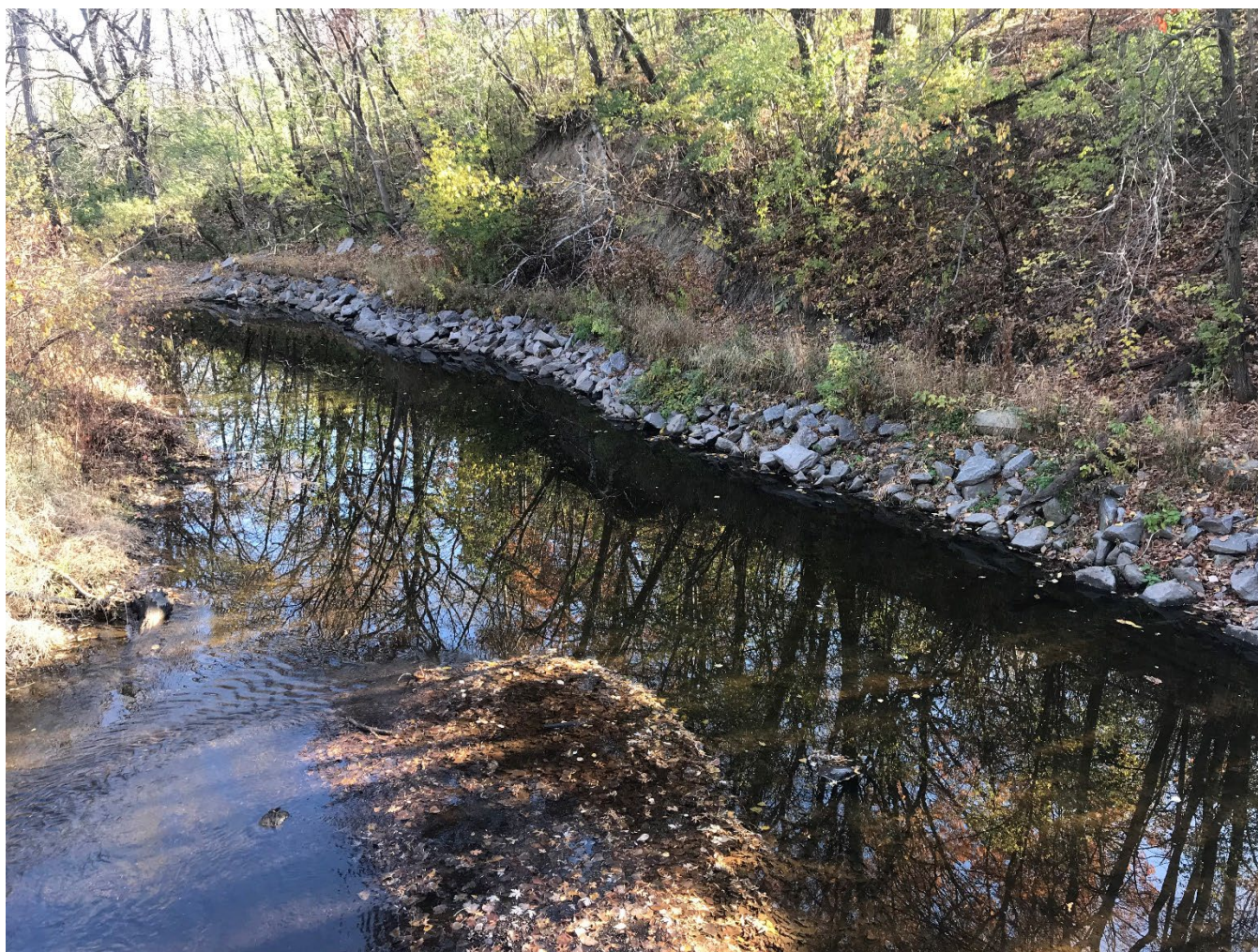
Figure 56. Stabilization Area 9 showing riprap toe and vegetated bench upstream of trail bridge. Photo taken on 10/28/2022.
