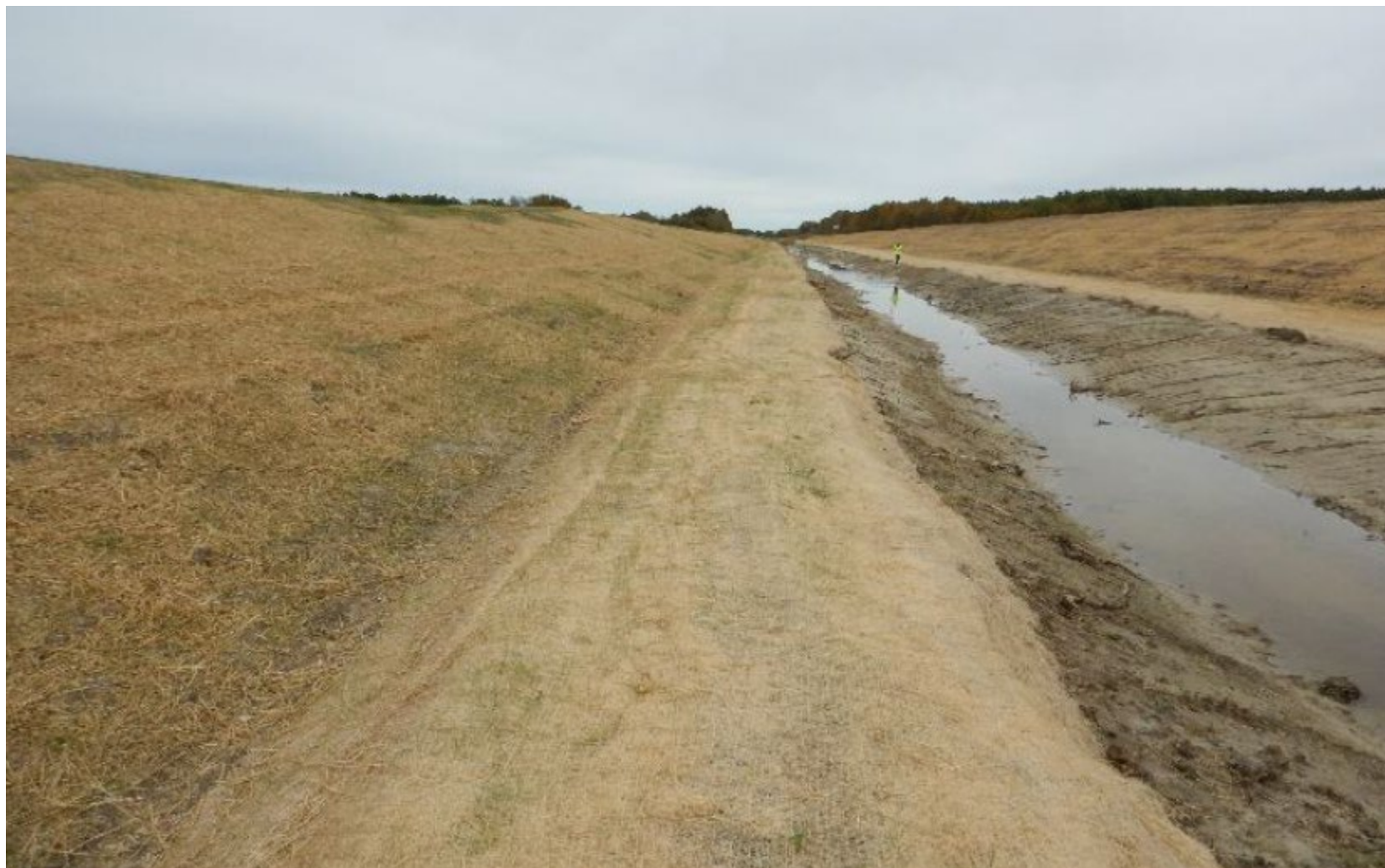
Photo 94. Construction photo looking east alongside bench of 2-stage ditch (Bostic Creek Grade Stabilization – photo from Project Summary PowerPoint).
