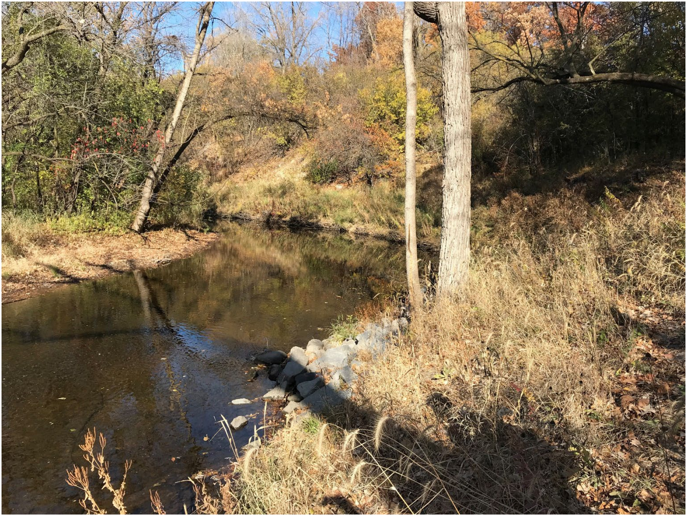
Figure 59. Stabilization Area 4 showing toewood and boulder rock vane at upstream terminus of the toewood structure. Photo taken on 10/28/2022.
