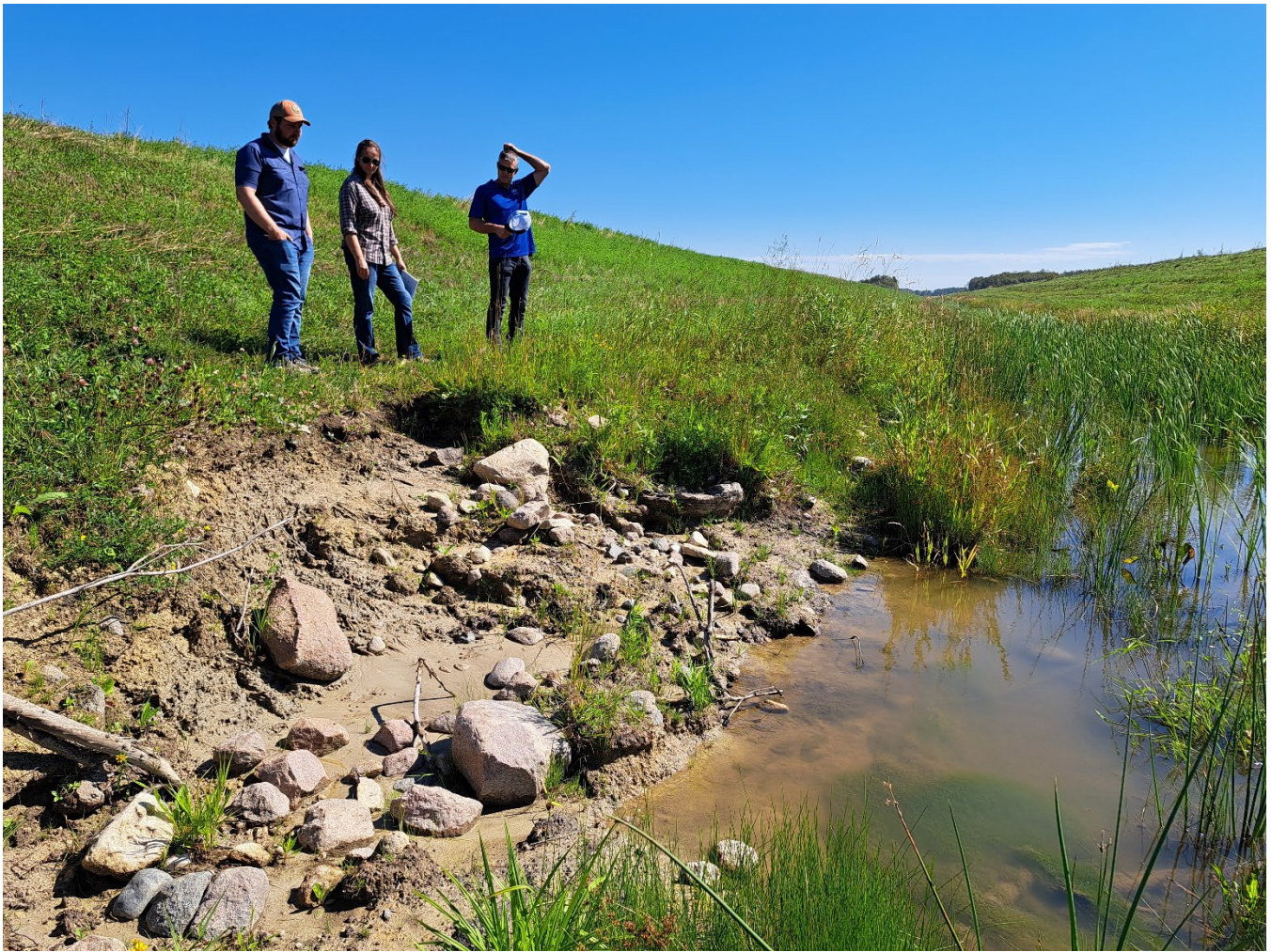
Photo 101. Looking east along 2-stage ditch where spring flooding cut into the bank (Bostic Creek Grade Stabilization, photo taken during site visit 8/30/2022).
