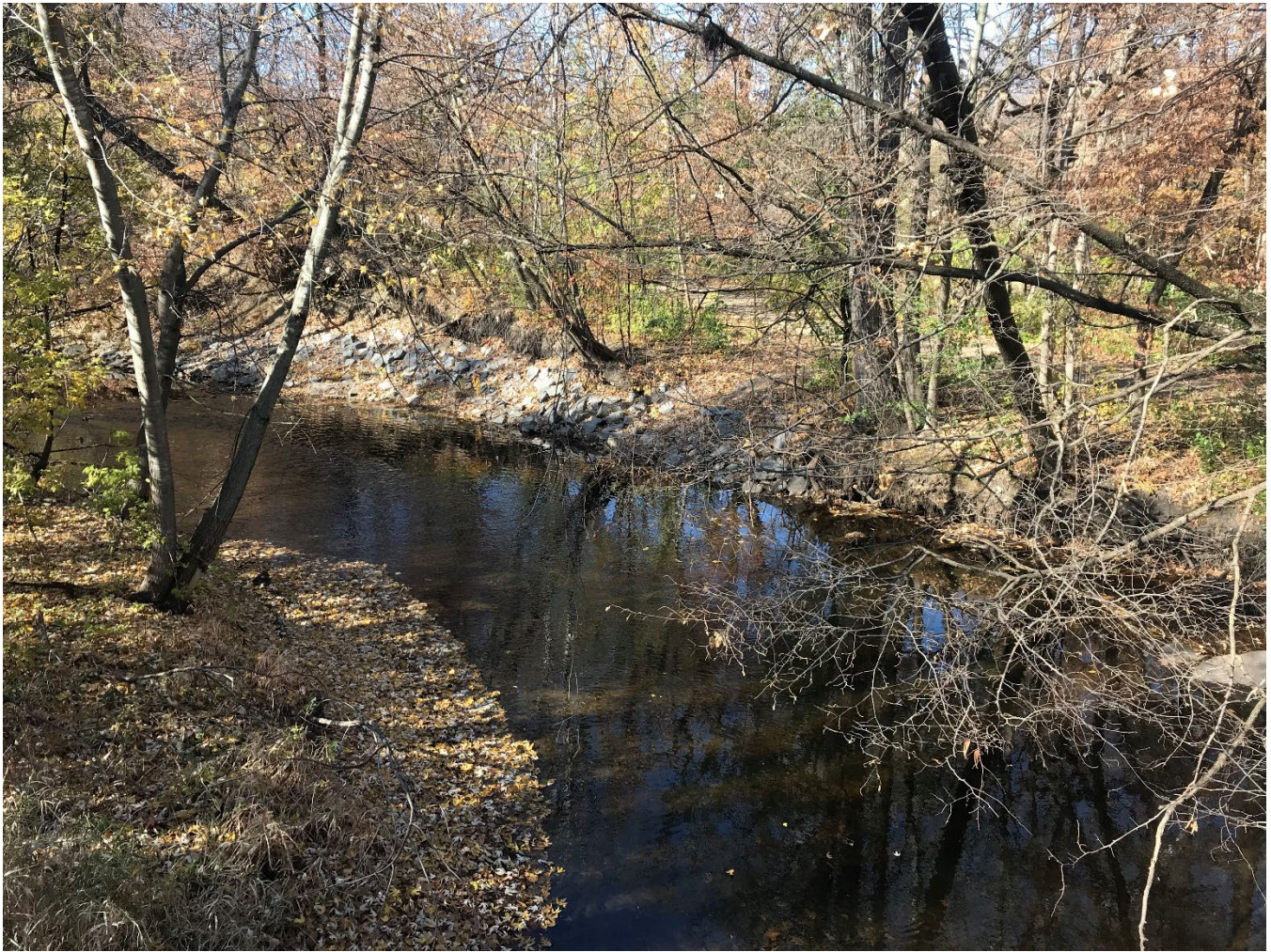
Figure 58. Stabilization Area 3 showing riprap along a previous cutbank. Photo taken on 10/28/2022.
