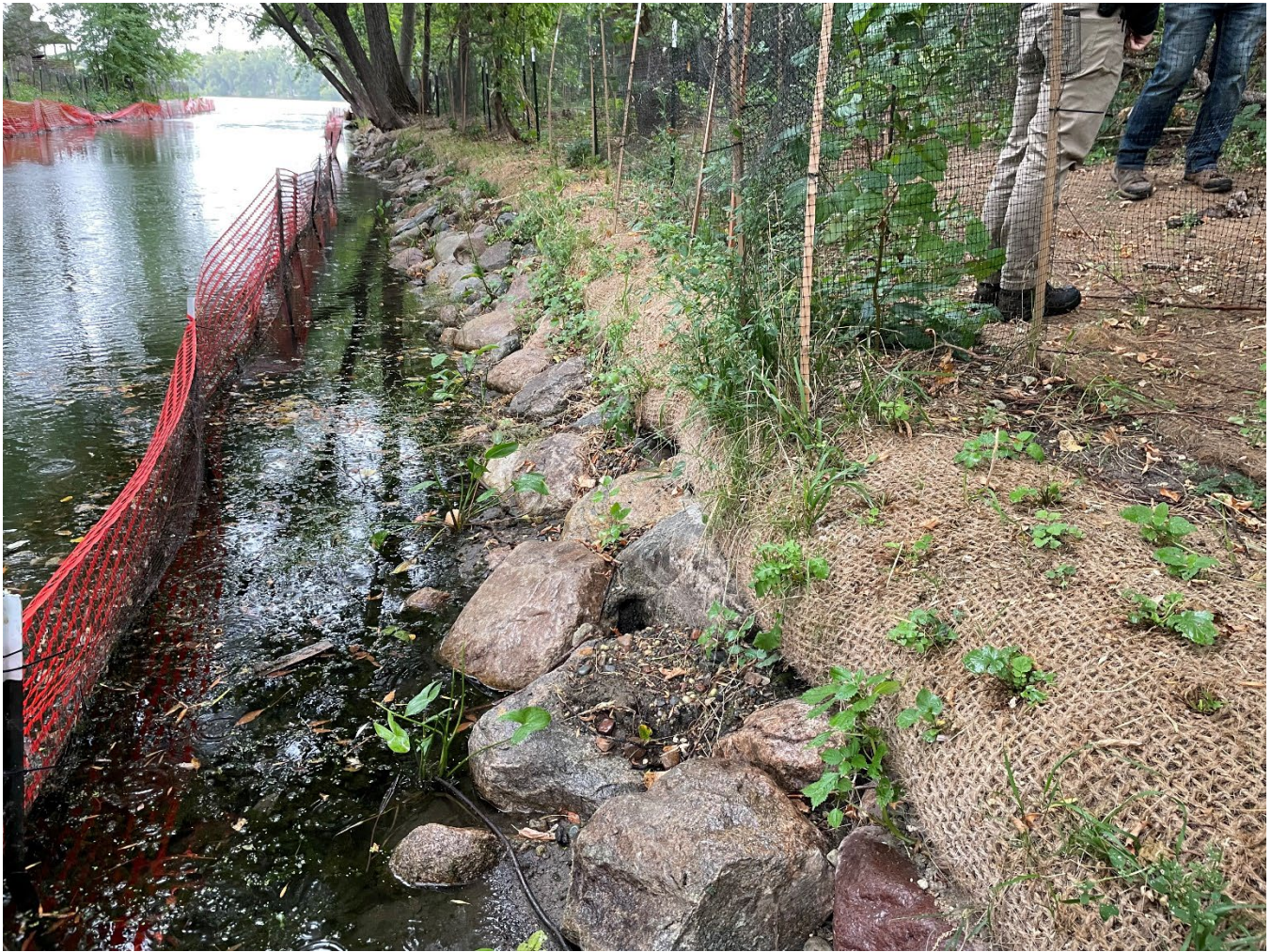
Photo 75. Looking to the northwest along Kenilworth Channel towards Cedar Lake outlet. Note the rocked toe as well as the FES (Fabric Encapsulated Soil) lifts alongside the channel (Kenilworth Channel Shoreline Stabilization, photo taken during site visit 9/23/2022).
