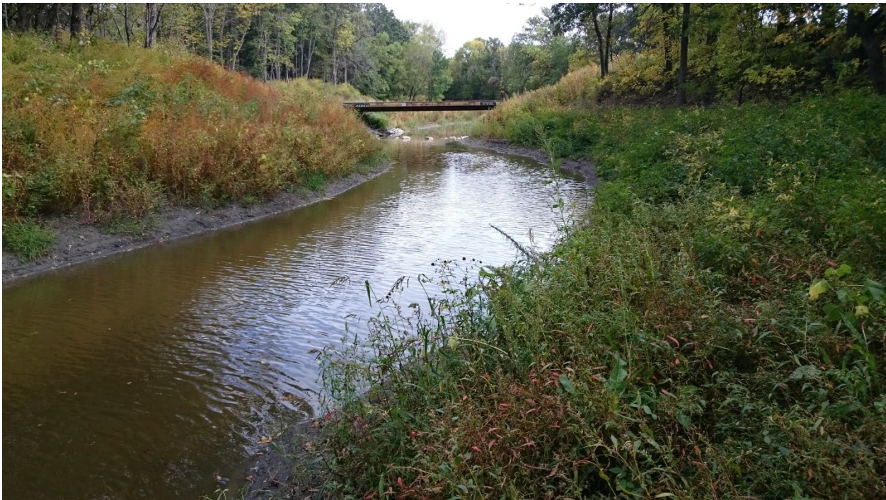
SR Photo 29: Channel graded in cleared woods.
