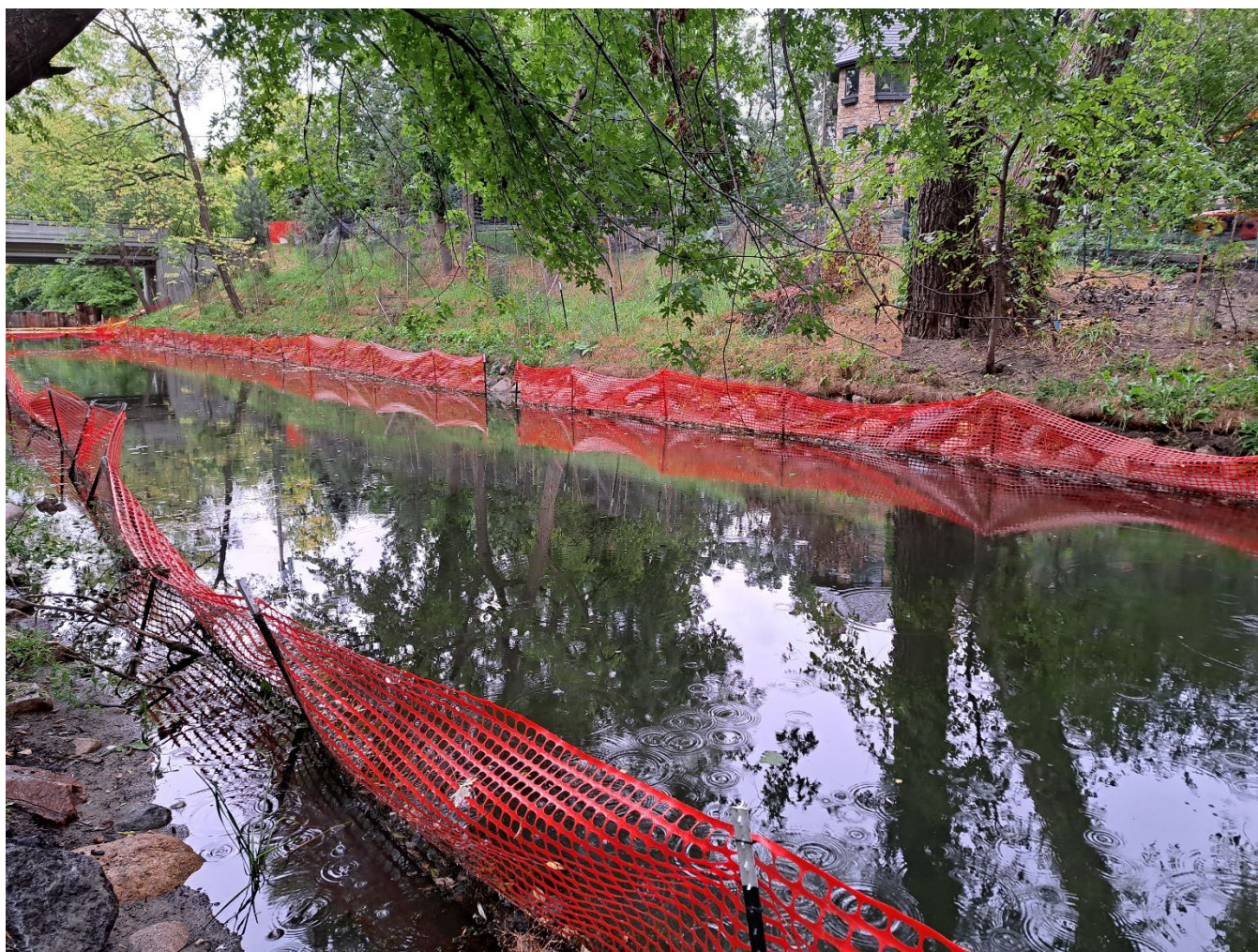
Photo 71. Looking to the southeast along Kenilworth Channel towards Burnham Road bridge. Note the snow fencing alongside the rocky toe to protect the native plantings from both geese and public disturbance (Kenilworth Channel Shoreline Stabilization, photo taken during site visit 9/23/2022).
