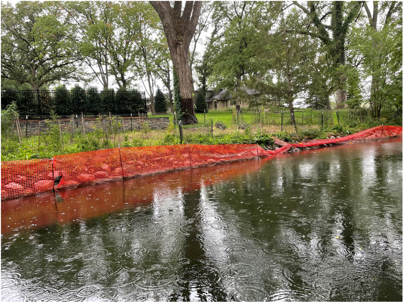
Photo 76. Looking to the southwest along Kenilworth Channel near the Cedar Lake outlet. Significant efforts by the project managers were undertaken to protect the native plantings including snow fencing along the channel as well as netting surrounding the trees and shrub planting (Kenilworth Channel Shoreline Stabilization, photo taken during site visit 9/23/2022).
