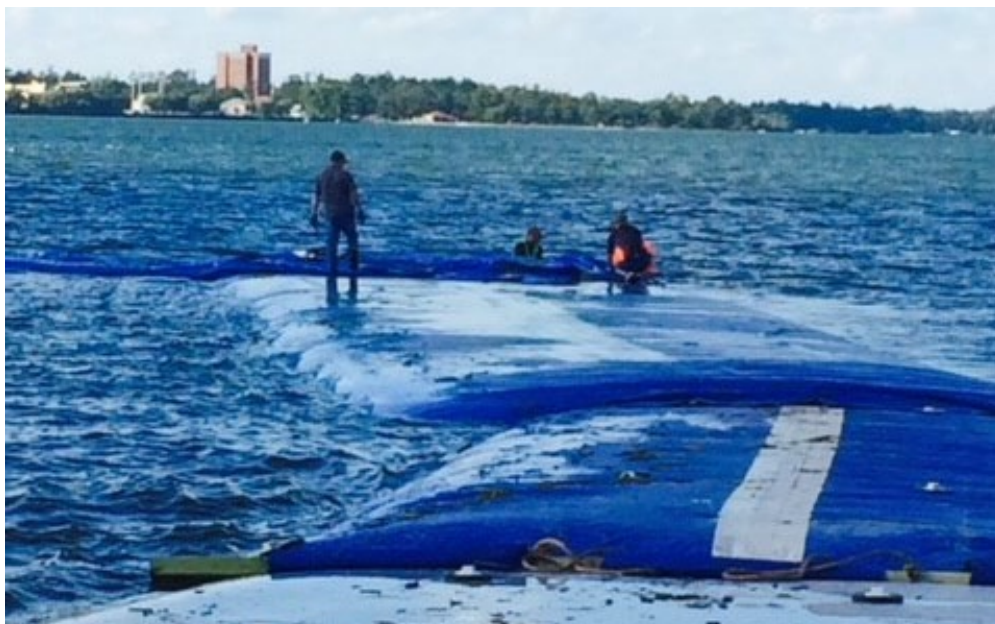
Photo 41. AquaBarrier® installation at Lake Bemidji prior to lake sediment dredging (Lake Bemidji South Shore Enhancement – photo from City of Bemidji).
