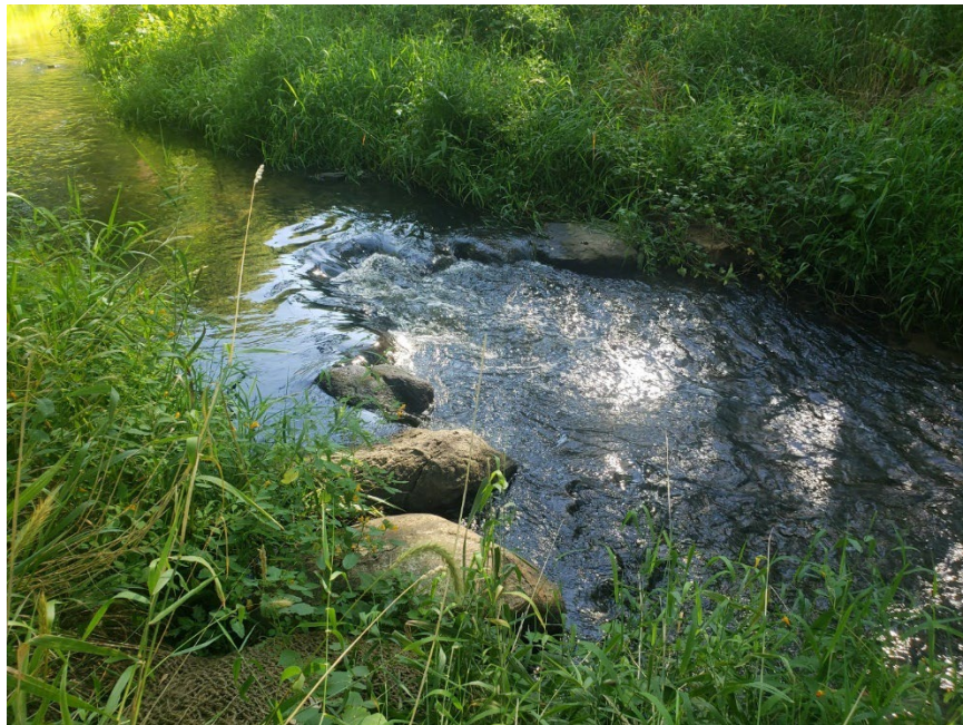
Photo 82. Example of stone grade control. The structure points upstream with the arms angled up and towards the bank to direct flows into the center of the channel and away from banks while providing grade control to the stream bed. (Photo taken by Mark Prankus, Cardno now Stantec, on 9/1/22).
