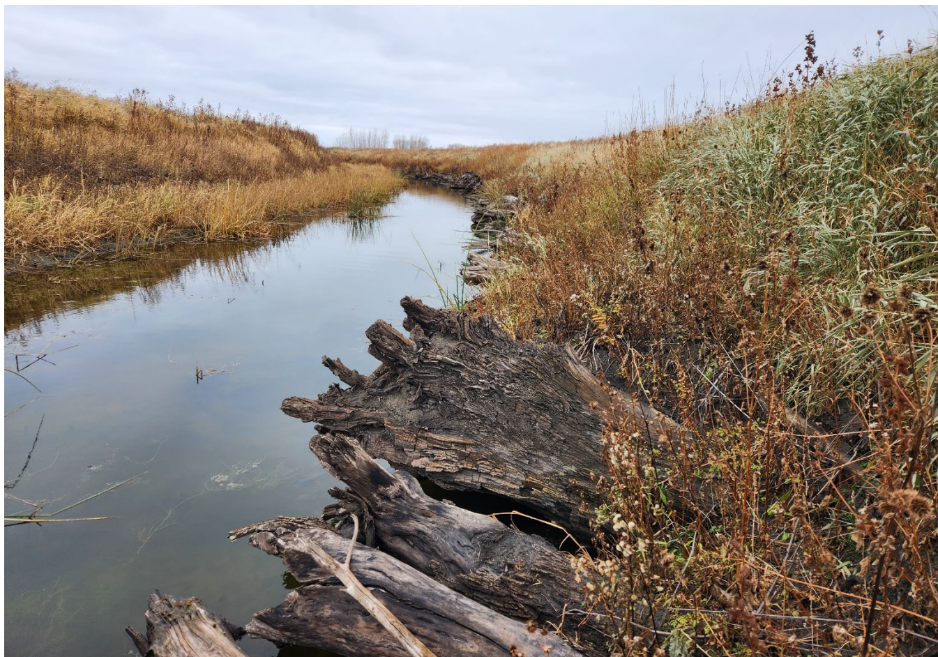
Photo 58. Toe wood installations along Grand Marais Creek. Photo taken on 10/25/2022.
