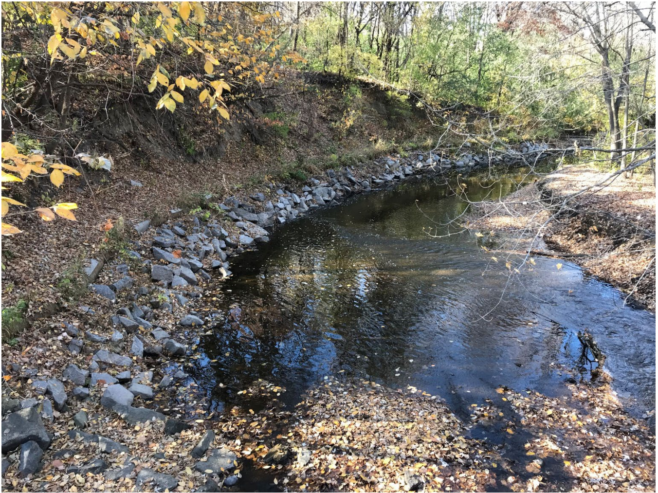
Figure 57. Stabilization Area 9 showing riprap toe and vegetated bench along cutbank downstream of trail bridge. Photo taken on 10/28/2022.
