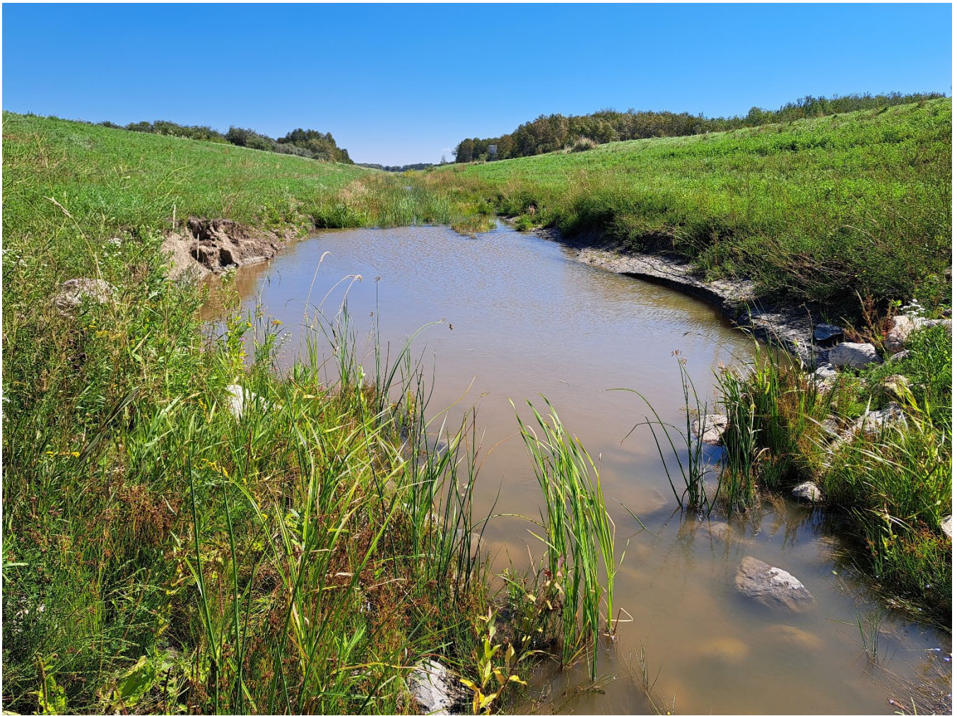
Photo 105. Looking east/downstream below failed riffle where scouring occurred during spring flooding (Bostic Creek Grade Stabilization, photo taken during site visit 8/30/2022).
