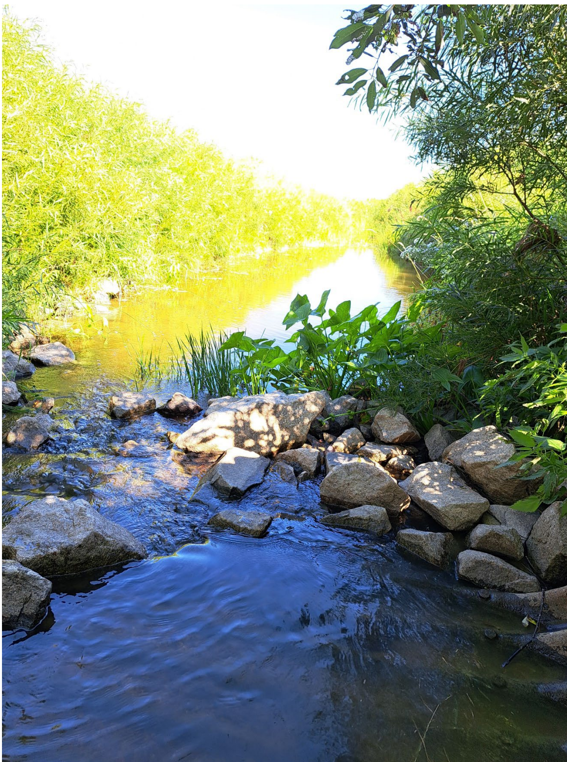
Photo 96. Looking north from County Hwy 4 (Graceton Beach Rd) at a rock bar installed downstream from a culvert (Bostic Creek Grade Stabilization, photo taken during site visit 8/30/2022).
