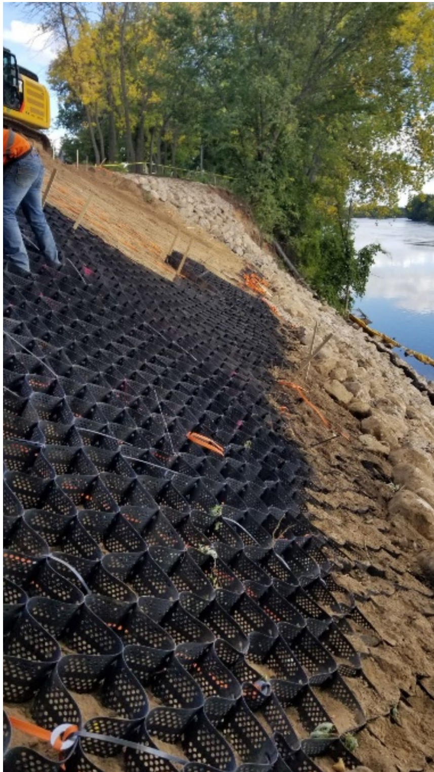
Photo 87. Example of the reinforced soil slope with in-situ soil bioengineering treatment during construction (Photo provided by Anoka County Conservation District, 9/16/2020).
