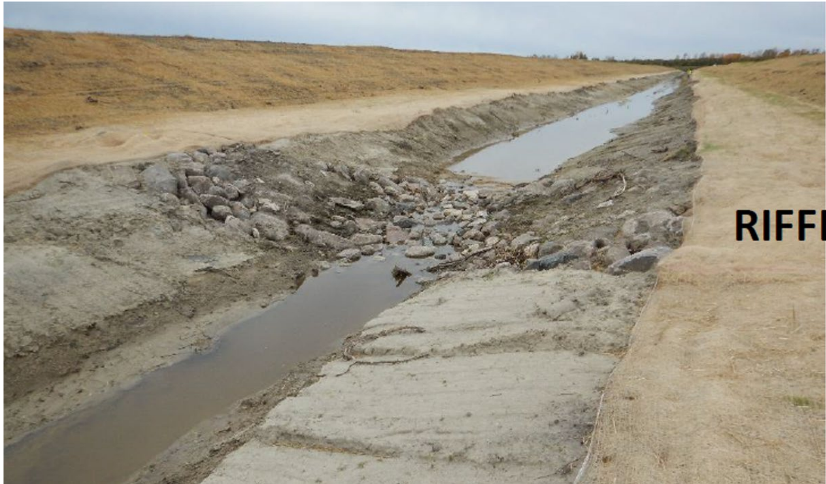
Photo 95. Riffle construction photo looking southwest (Bostic Creek Grade Stabilization – photo from Project Summary PowerPoint)
