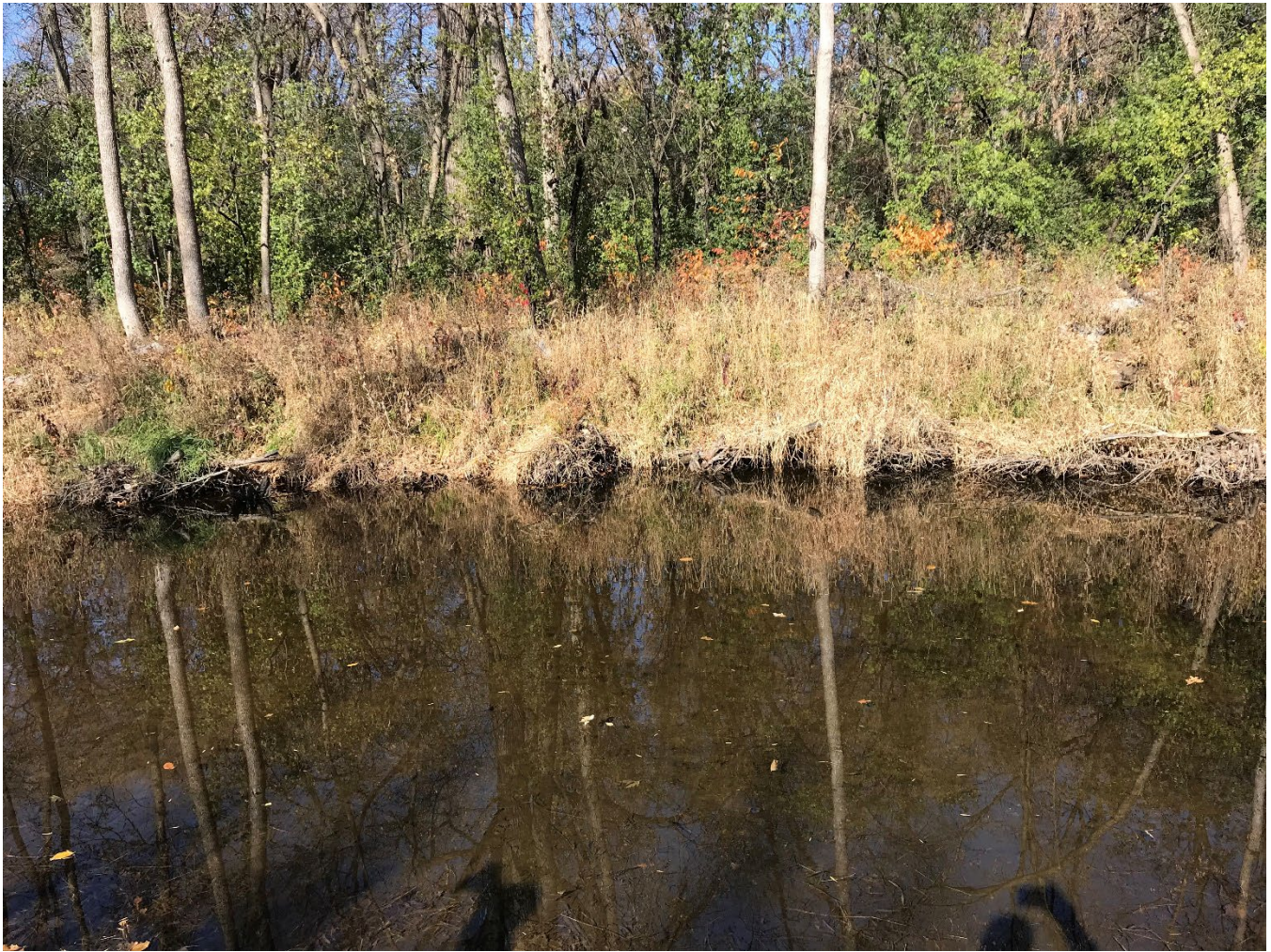
Figure 63. Stabilization Area 12 showing toewood and three soil lifts installed above the toewood structure. Photo taken on 10/28/2022.
