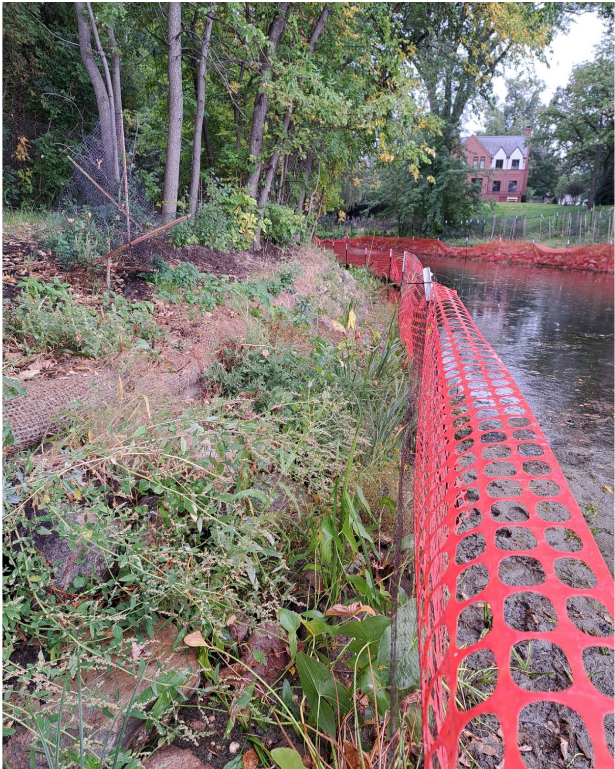
Photo 74. Looking towards Kenilworth Channel at the outlet location of Cedar Lake. Note the presence of planted emergent plugs such as arrowhead, prairie cordgrass and sweet flag (Kenilworth Channel Shoreline Stabilization, photo taken during site visit 9/23/2022).
