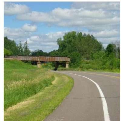
County Highway 61 curves under the St. Croix Valley Railroad north of Rock Creek.
