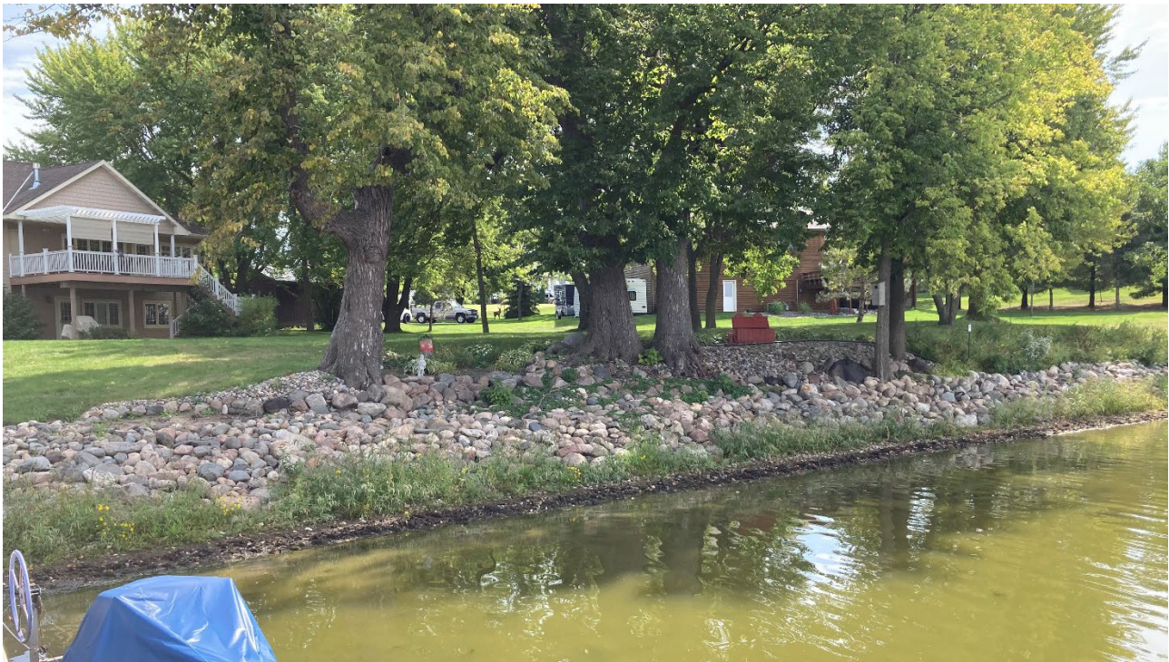
Photo 8 Completed project viewed from the water during site visit 09/13/2021.
