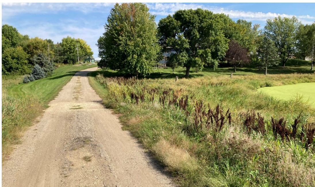
Photo 12 Looking north where new culvert crosses under driveway in center left of photo. This new culvert connects runoff from the upper watershed to the wetland basin on the right.
