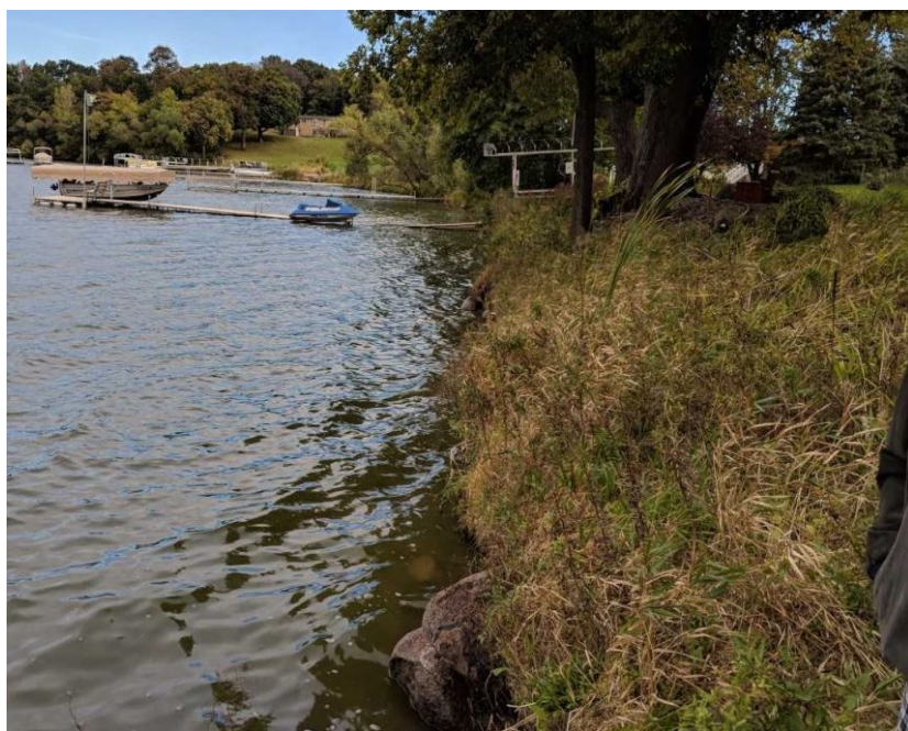
Photo 6 Pre-project photo of shoreline looking north 2019. Project manager reported that the toe was continually eroding and beginning to undercut the roots of existing Basswood trees.
