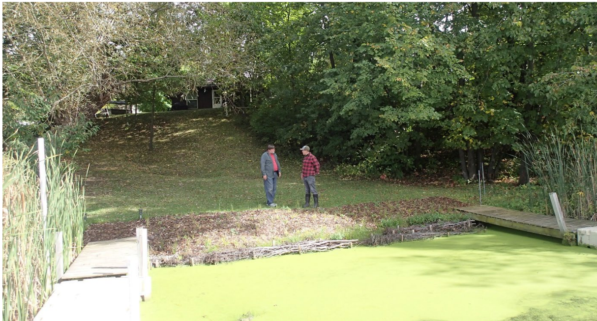
Photo 24 Project site with willow wattles at shoreline and buffer planting above.
