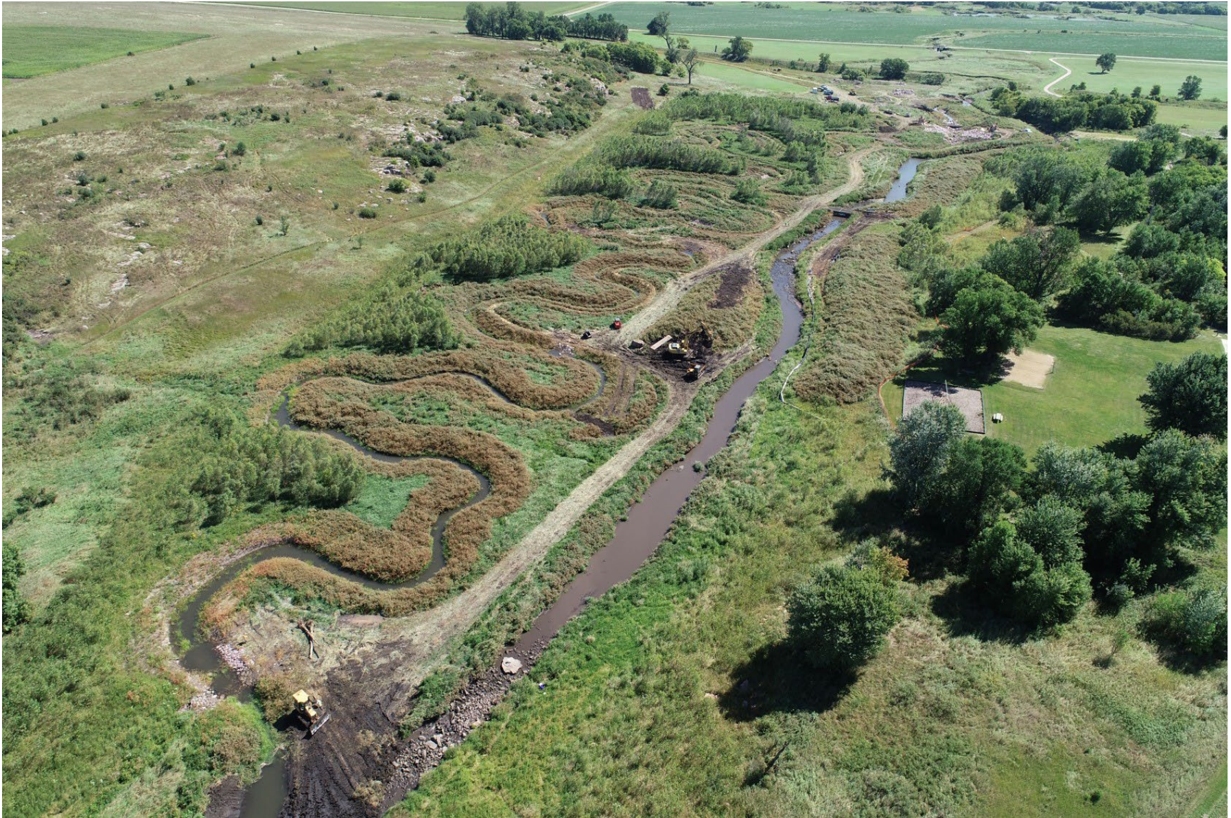
Photo 7-9. Aerial view of the project area just before moving water into the new channel.
