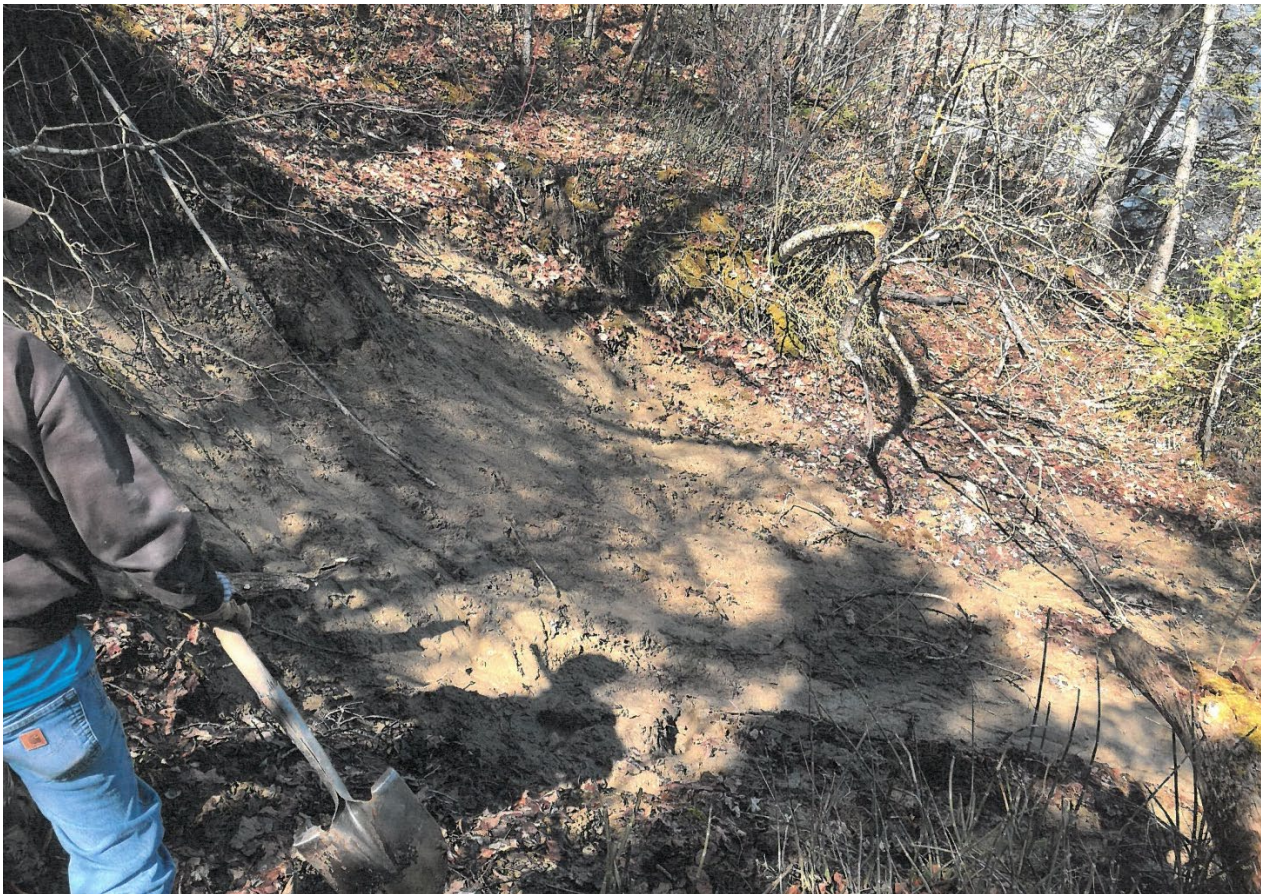
Photo 39 Site Conditions immediately prior to installation.
