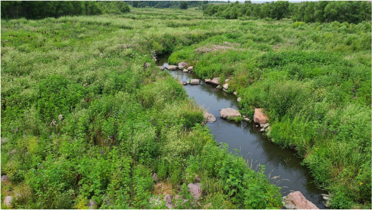
Photo 7-1 Blue Mounds State Park, photo taken during site visit 07/26/2021. Looking upstream at Mound Creek reconstructed channel and floodplain with contractor seeding to left (south bank).
