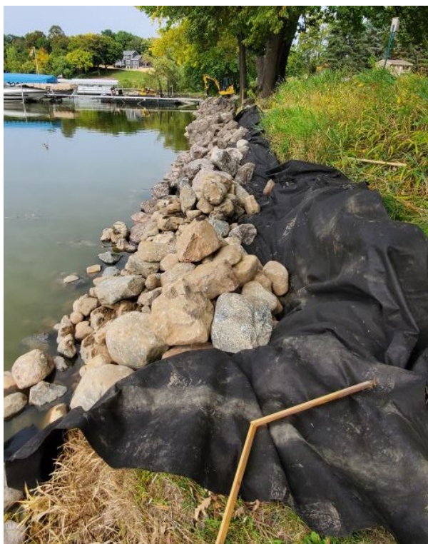
Photo 7 Site photo during construction facing north 2020.
