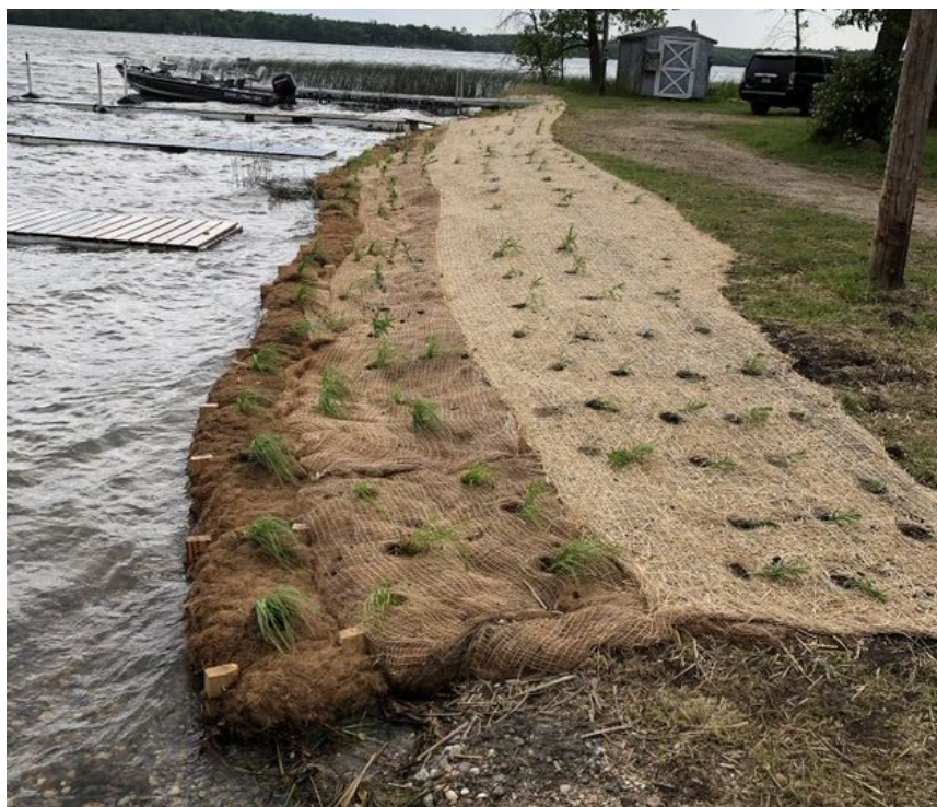
Photo 33 Biolog, coconut fiber blanket and plug plantings installed, summer 2021.
