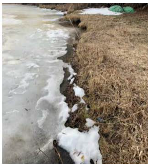
Completed Project Site Photo
