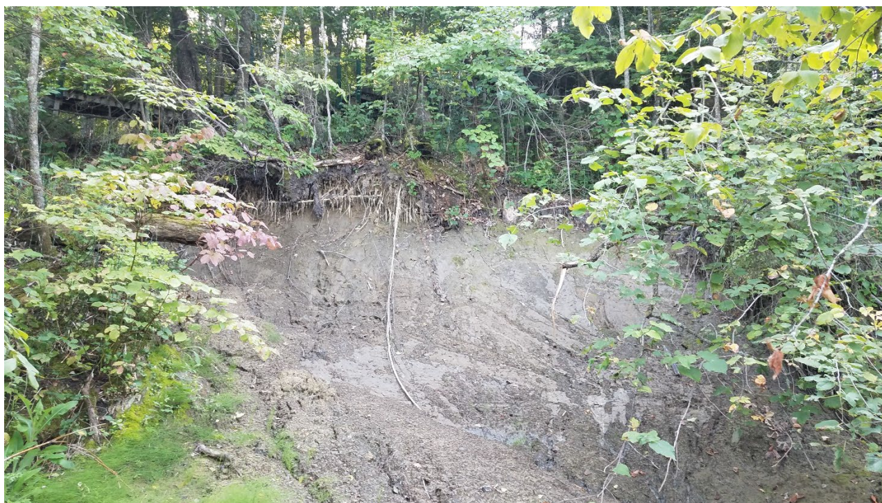
Photo 36 Top of sluffing slope pre-project 2019.
