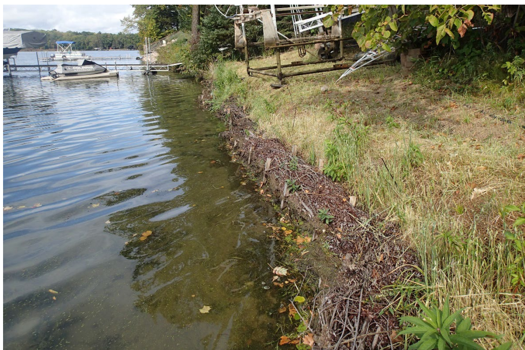
Photo 22 Willow wattle anchored to the shoreline toe and seeded and planted vegetation beginning to grow along buffer.
