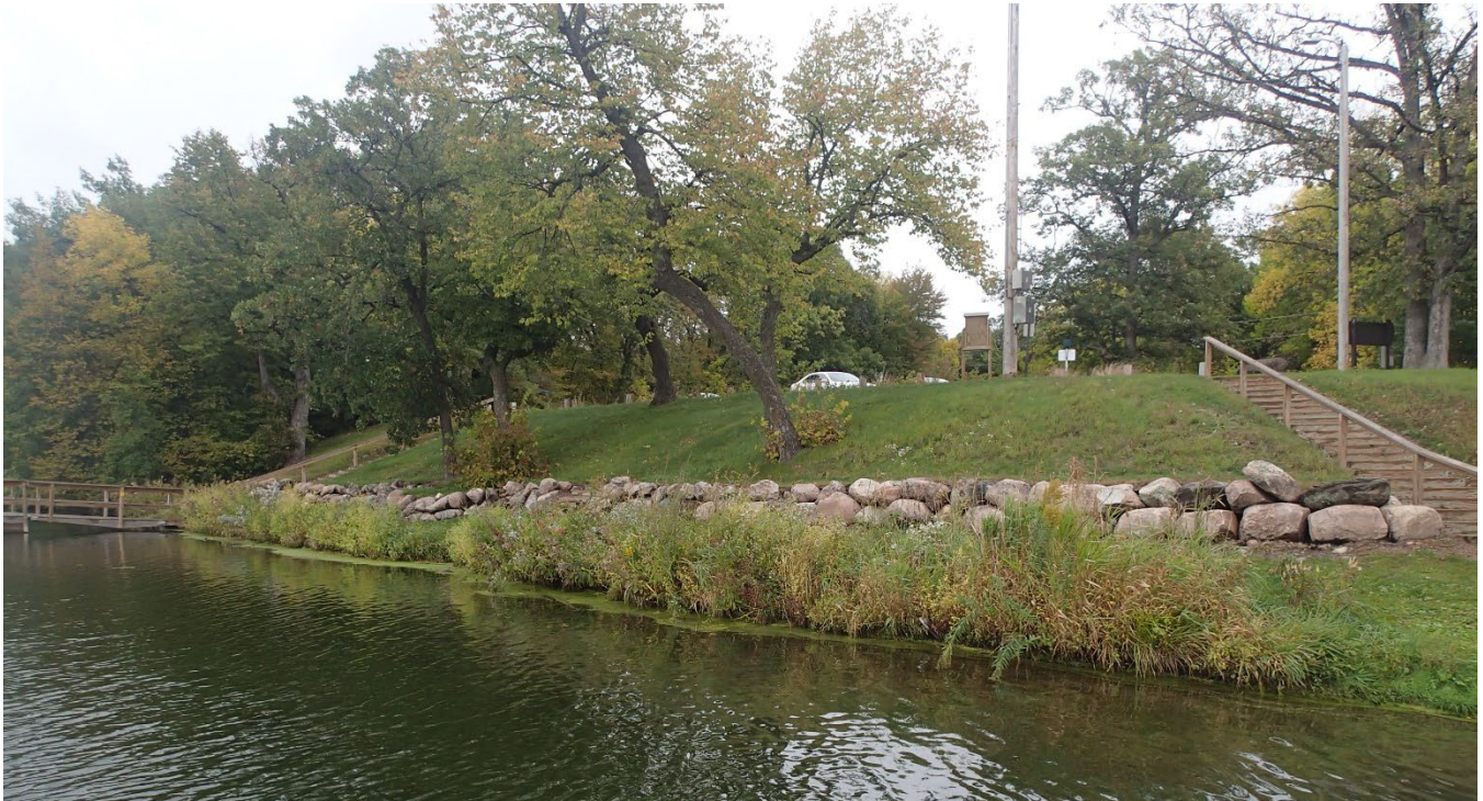
Photo 20 Slope and planted shoreline buffer. Installed biologs at the shoreline toe are secure and well vegetated with plant roots. Photo from site visit 09/24/2021.
