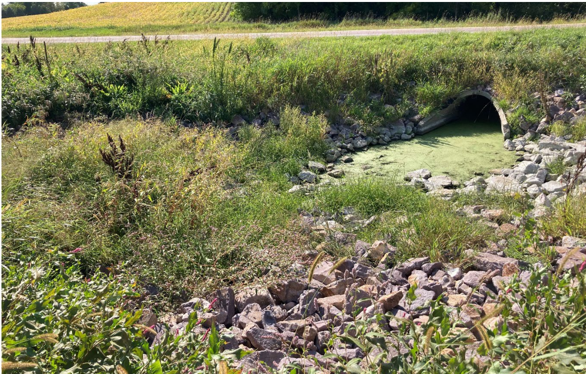
Photo 15 Riprap outlet at southwest corner of wetland basin leading to road culvert. Standing water with duckweed in culvert is the result of recent rains prior to site visit. Plan detail shown figure 4
