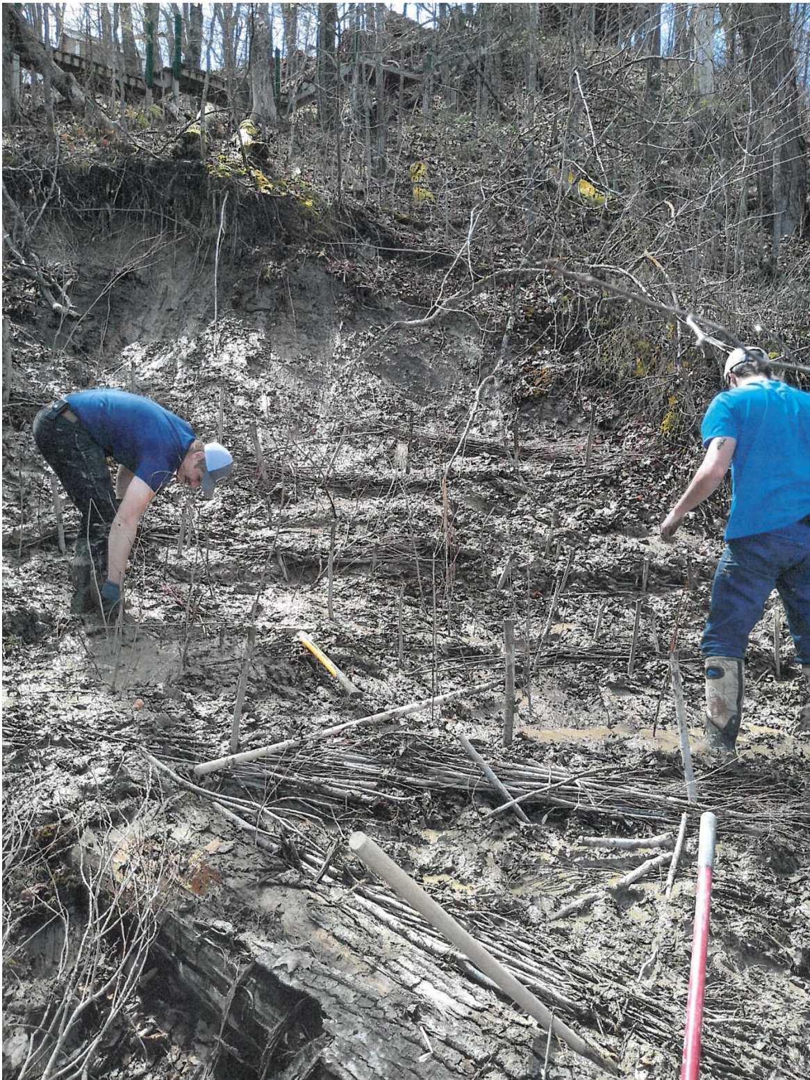
Photo 40 Installation of fascines and live stakes, April 2020.
