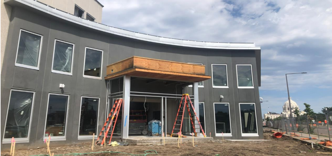
Photo of St. Paul City School under construction along University Avenue. CAAPB worked closely with school leadership and architects on planning, design, and approval. (Credit: Peter Musty)
