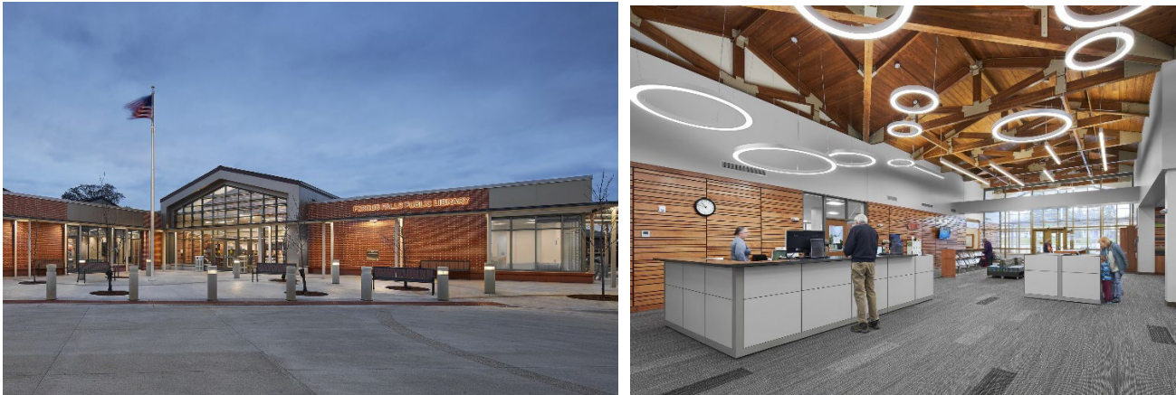
Figure 9(left) & 10(right). Fergus Falls Public Library: 25,600 sf building in Fergus Falls. Annual savings over code are estimated at 1,234 mmBtu, $22,779 and 65 tons of carbon.
