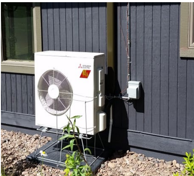
Figure 5. Ductless Cold-Climate Air-Source Heat Pump, which Includes an Outdoor Condenser Unit (left) and an Indoor Evaporator Unit or Head (right). (Photos courtesy of the Center for Energy and Environment)
