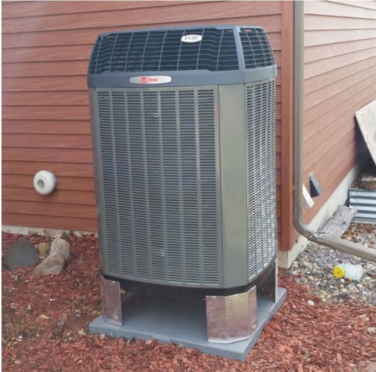
Figure 5. Ductless Cold-Climate Air-Source Heat Pump, which Includes an Outdoor Condenser Unit (left) and an Indoor Evaporator Unit or Head (right). (Photos courtesy of the Center for Energy and Environment)
