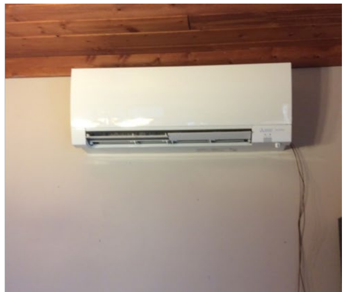
Figure 5. Ductless Cold-Climate Air-Source Heat Pump, which Includes an Outdoor Condenser Unit (left) and an Indoor Evaporator Unit or Head (right). (Photos courtesy of the Center for Energy and Environment)
