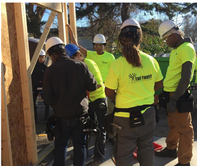
Tree Trust Youthbuild framing a house
