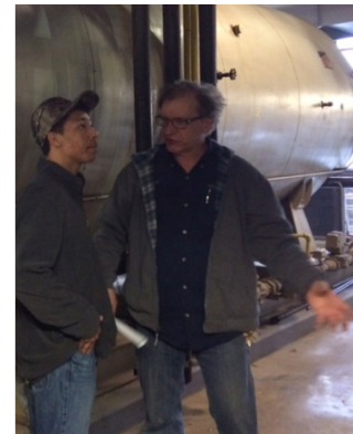
Kaleb during a Tour and demonstration of boiler systems.
