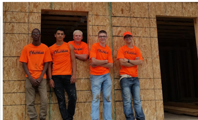
Career Solutions crew at a Habitat for Humanity home.
