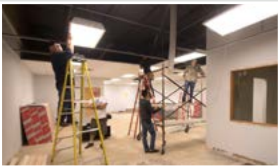
SouthWest Metro construction project
