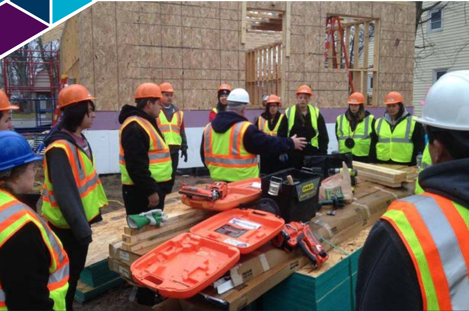
BICAP Youthbuilders construct an affordable home in Bemidji.
