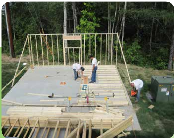
AEOA youth constructing a garage.
