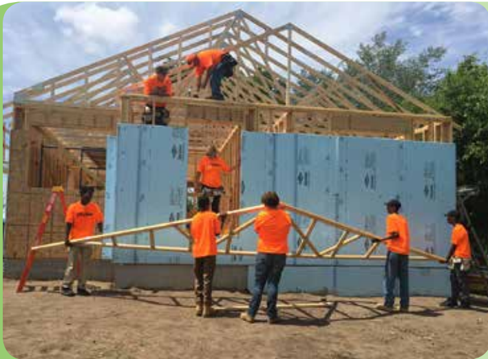
Youthbuilder adding trusses to a Habitat for Humanity home.
