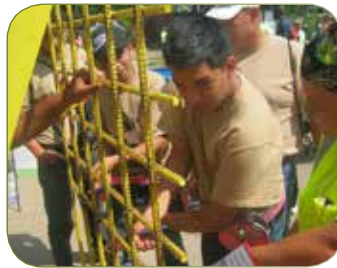
Youthbuilders tying rods at Construct Tomorrow Event.
