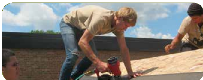
Roofing a shed for Habitat for Humanity.
