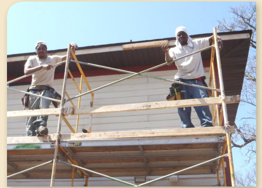
Creston and Jeremy on scaffolding.
