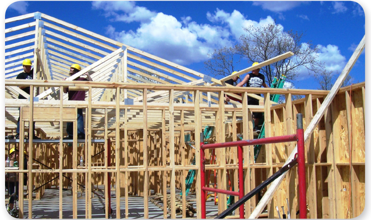
Kyle, Richard, and Joe install trusses with Bi-CAP Intern, Taylor.
