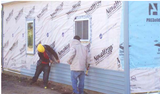
Rickard and Kyle apply vinyl siding to a MURL house.
