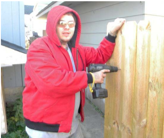
Miles erects a new fence at a renovated home in Eveleth.
