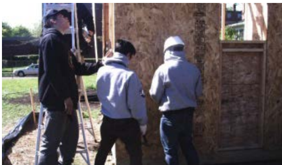
GAP Youthbuilders constructing a utility shed in St. Paul.
