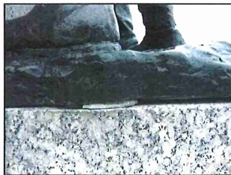
Grout needs to be redone at base of sculpture.
