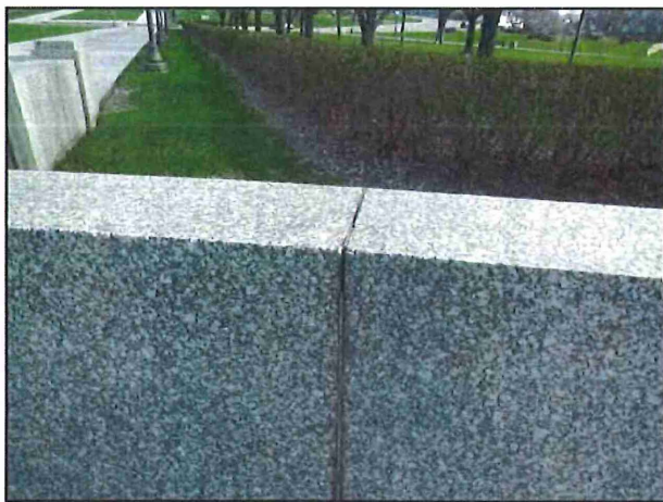
Grout joints need to be reworked along with conservation of all plaques.
