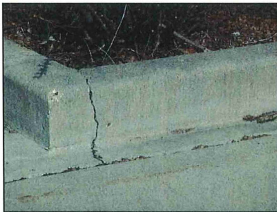
New concrete curb surround should be constructed.
