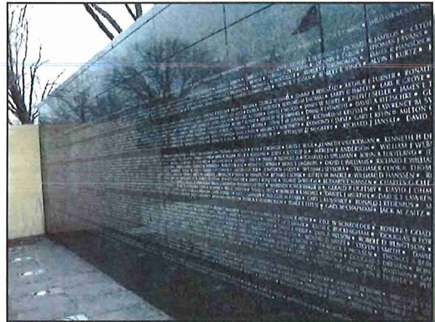
Failed ground lighting needs replacement with overhead wall wash lighting.
