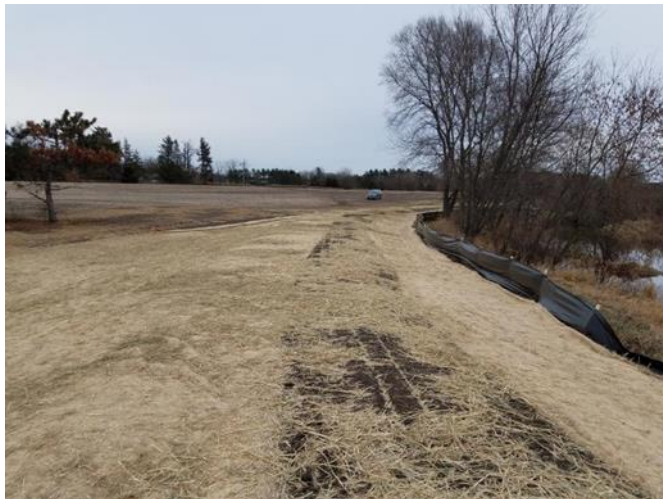
Figure 5. Grade stabilization structure helped reduce erosion
