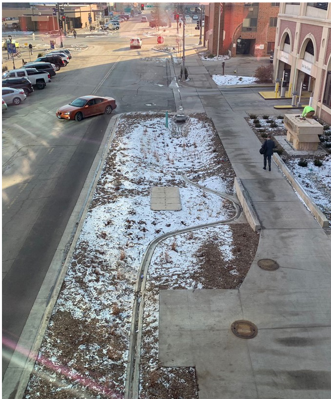
Overview of nearly completed demo stormwater system.
