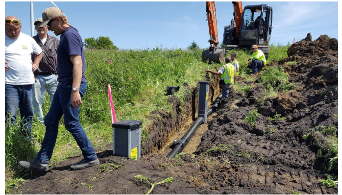
Saturated buffer construction at Tapp Farm
