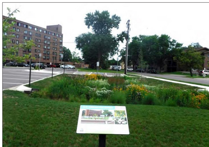
Rain garden project installation
