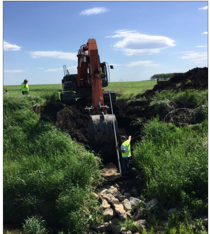
Greater Blue Earth River Basin ditch area drainage project
