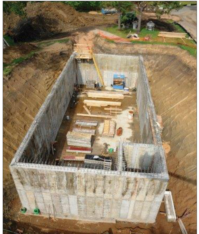
Northwoods tank construction
