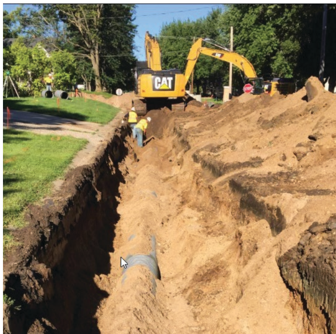
Street reconstruction project
