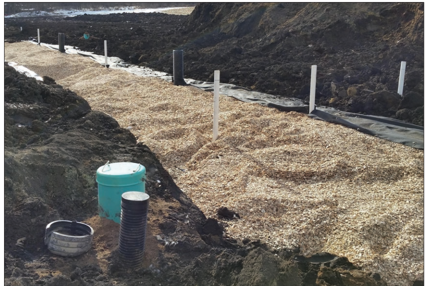
County Ditch 62 watershed construction
