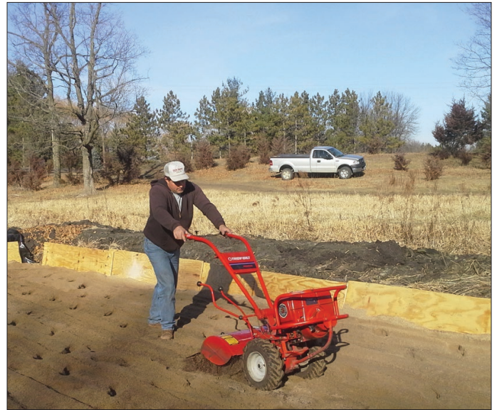
Construction iron aggregate being mixed with sand by rototiller
