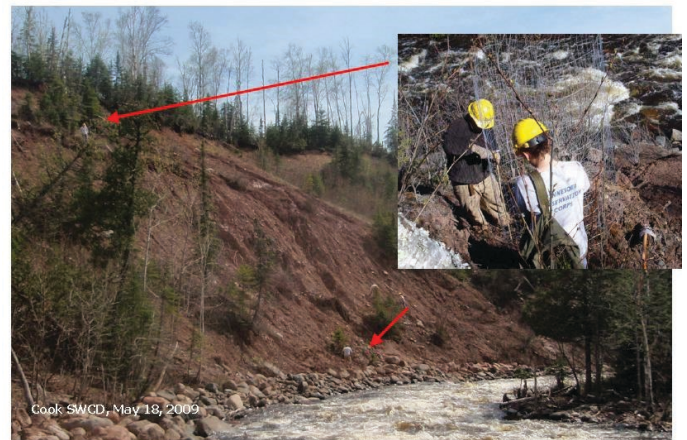
MIN Conservation Corps crews planting trees, shrubs, and grasses on the stabilized slump, with the expectation they will spread over the bank and reduce erosion from wind and raindrops.
