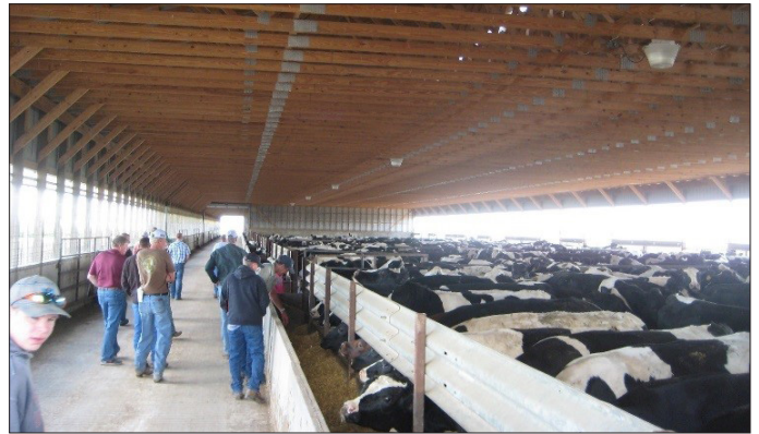
Dairy-beef covered feeding facility with slotted floors and pit manure storage.
