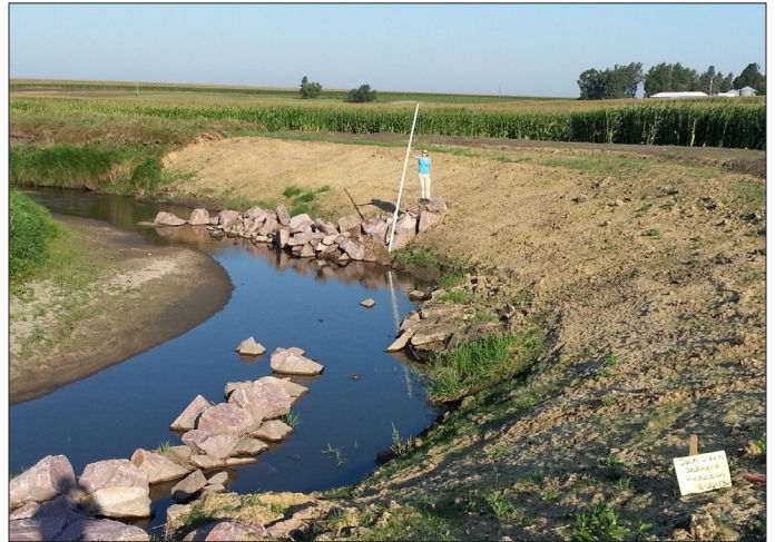
Jack Creek J-hook weir project, Section 34, Graham Lakes Township, Nobles County
