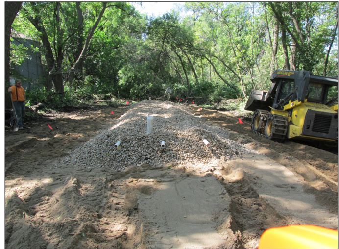
Mound system installation, NE ¼ of Section 34, Bondin Township, Murray County
