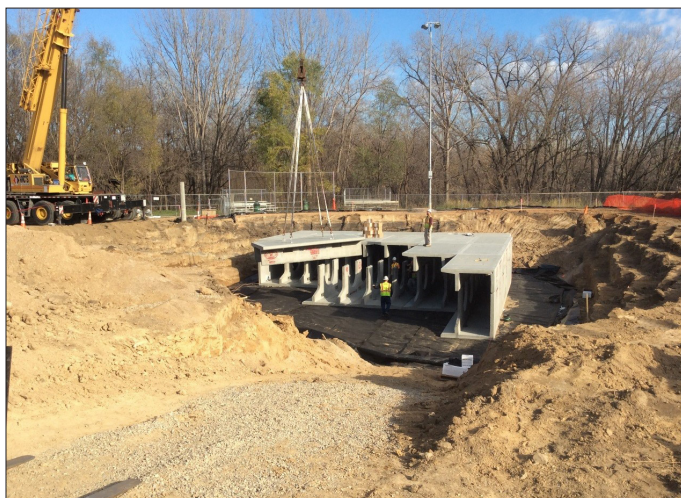
Modular Concrete Cistern Installation
