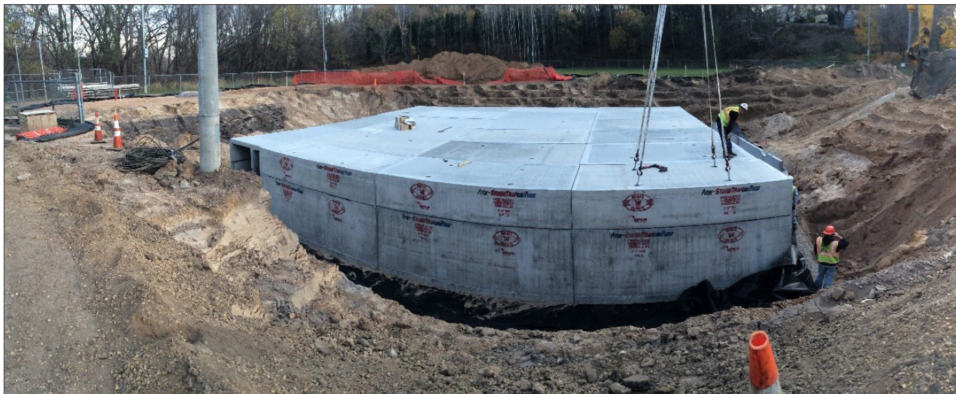
Installation of the Final Cistern Segment
