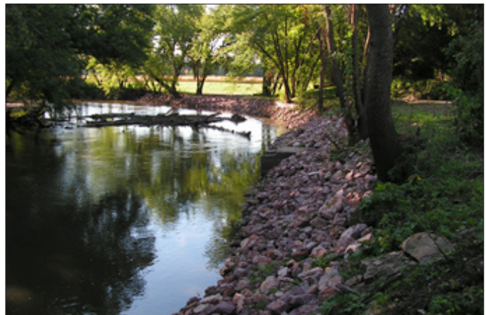
City of Springfield – Streambank Stabilization (2016)
