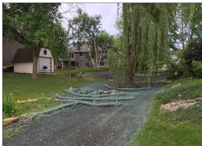
Channel stabilization in progress with erosion control
