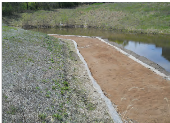
Assessing iron enhanced filtration trenches
