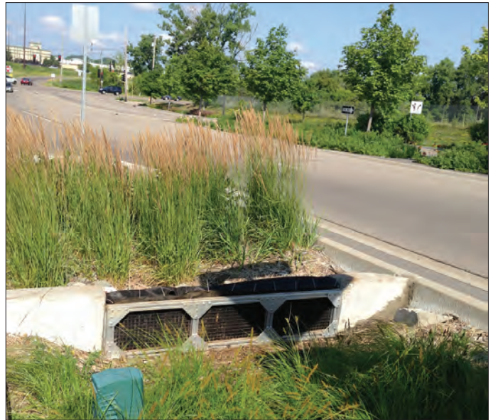
Photograph of the iron-enhanced ditch check installed at the City of Roseville swales.
