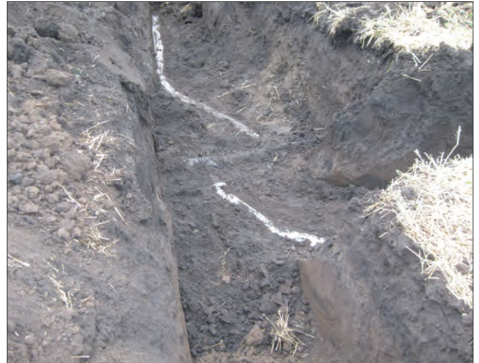
Wildung field day photo: Open tile intake replaced with pattern tiling
