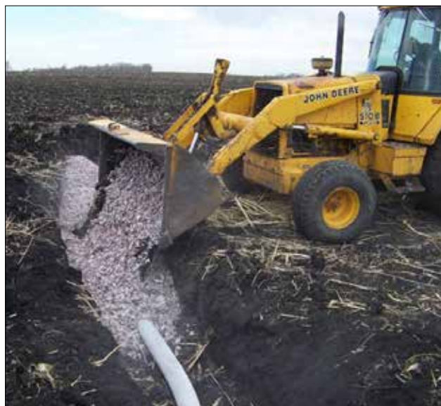
Rock tile inlet installation
