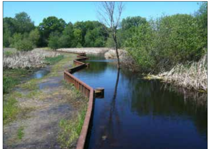
New outlet weir
