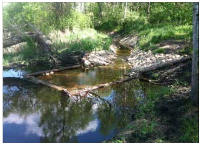
New overflow weir
