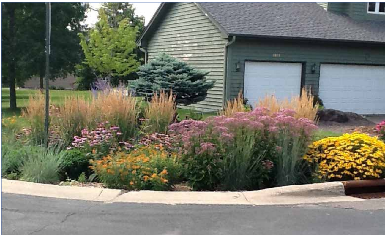
Rain Garden at the corner of Woodlawn Circle and Dunsmore Drive in Waconia, Minnesota
