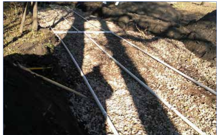
New septic system trench being prepared in Watonwan County
