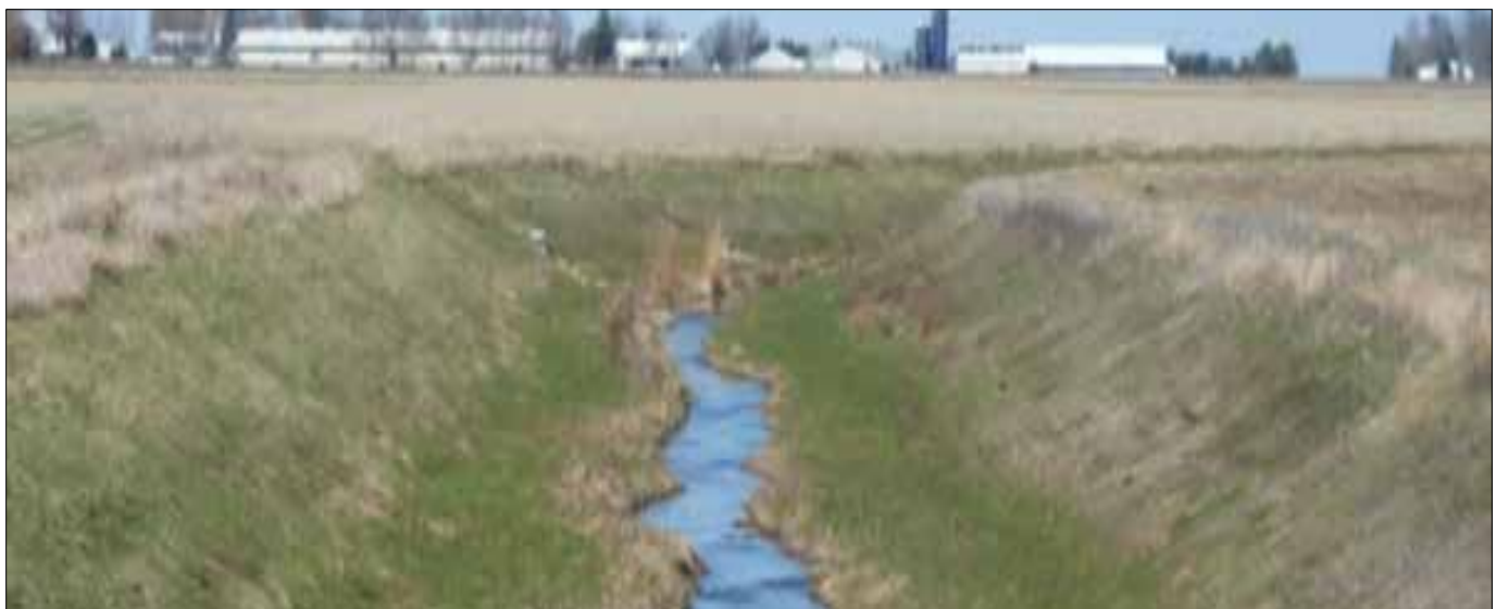
Two stage Mullenbach drainage ditch in Mower County, Minnesota
