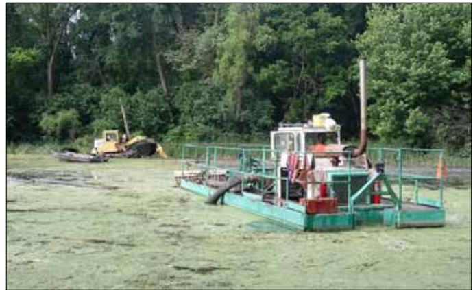
Villa Park 2013 dredging
