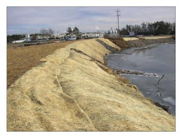
Long Prairie River, HWY 10 Motley, MN. Six stream barbs and rock riprap were used to stabilize the eroding bank that was threatening HWY 10.
