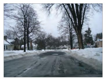
Abbott Avenue North looking south toward 41<sup>st</sup> Avenue North, ice-free section is porous asphalt and section with ice cover is traditional asphalt pavement.
