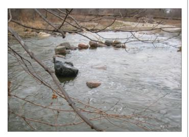
A close-up of the j-hook stabilization method utilized in the bank restoration project on the Redwood River near Lynd, Lyon County. J-hooks are positioned in such a way to provide a deep pool habit at the point of the hook while redirecting stream flow to inhibit bank erosion downstream.
