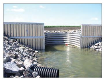
Meeker County, six foot aluminum drop structure at the head of a private ditch to control gully erosion and bank erosion.
