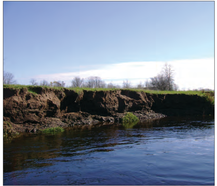
Shows some of the streambank erosion issues that are taking place along the lower parts of the Ann River. Sediment has been identified as a major contributor to the Fish and Invertebrate impairments in the Ann River.
