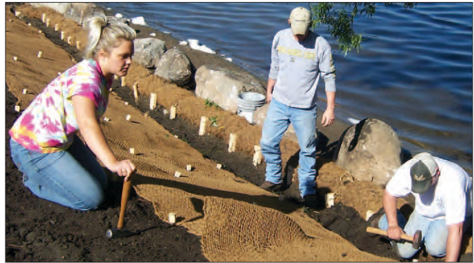
Lubben shoreline restoration project
