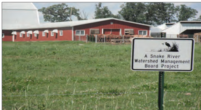
The picture is a site where a manure management system went in.
