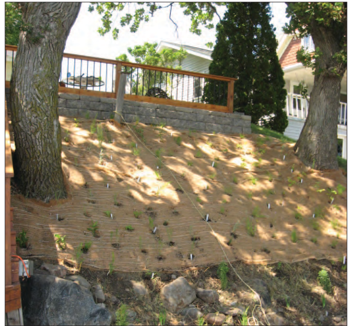
Shoreline stabilization project on Lake Florida
