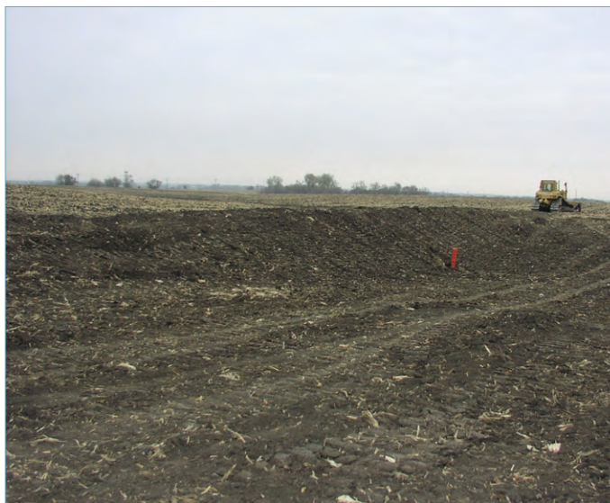
Yellow Medicine River Watershed – installation of a two acre waterway
