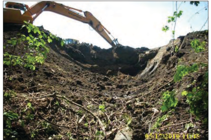
Installation of ravine stabilization structure in Seven Mile Creek Watershed
