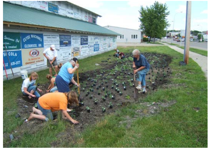
Rain garden construction at the Pope County Fairgrounds.
