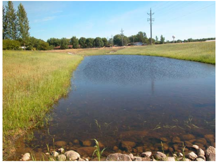
Stormwater retention project in the city of Osakis.
