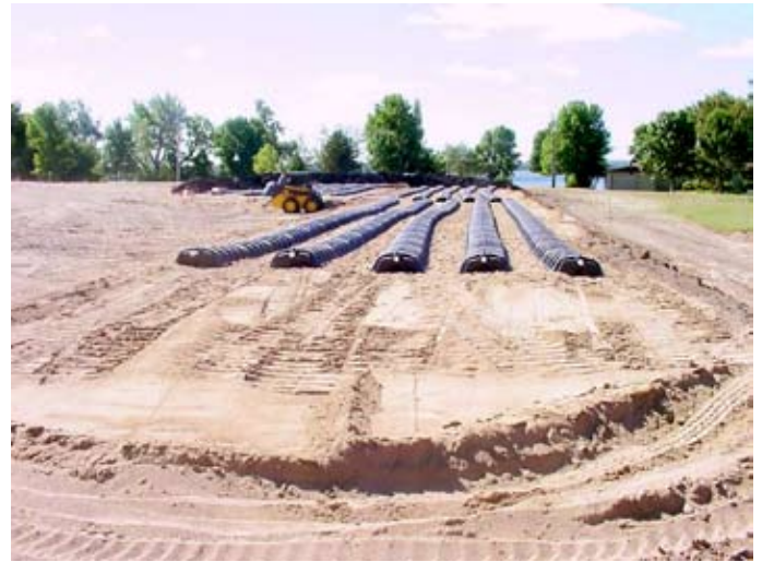
Installation of a septic system in Lincoln county.
