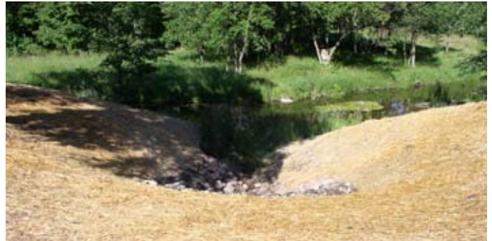
Gully erosion to Sauk River: before (top) and after (bottom).
