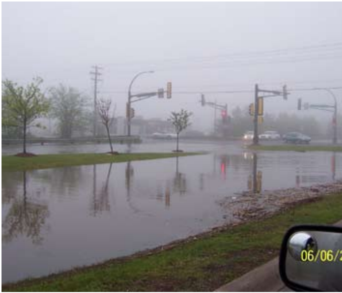
Miller Creek flooding during a storm June 6, 2008.
