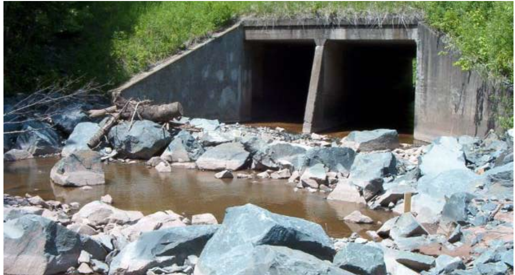
Highway 23 road culvert project.
