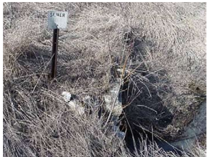
Community straight pipe into the stream at the small town of Taopi. All the systems in this town are now compliant and sewage no longer flows through this pipe.
