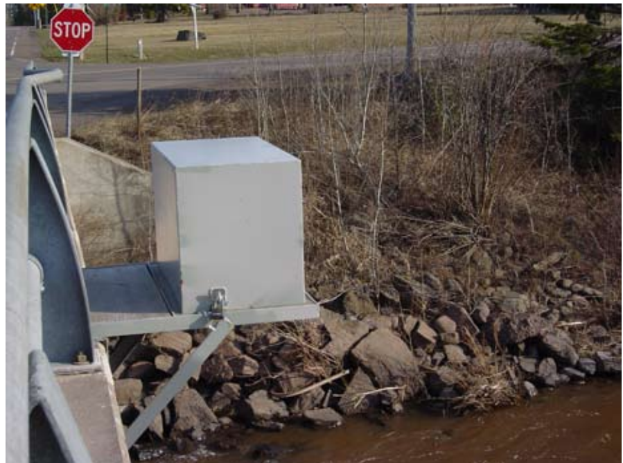
Box sampler installation at Knife River, near Knife River, MN.
