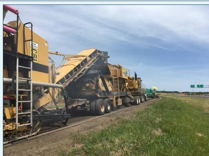
📷 Multi-unit CIR train milling and crushing an asphalt pavement
