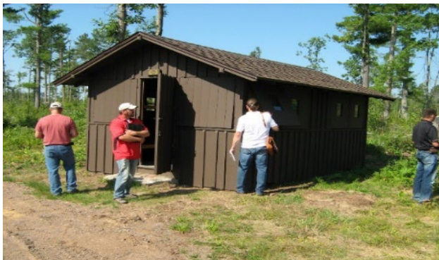
Figure 26: The St. John's Landing Group Camp Cabin in St. Croix State Park, one of many buildings that was damaged and repaired after straight-line winds on July 1, 2011. Photos by MN DNR
