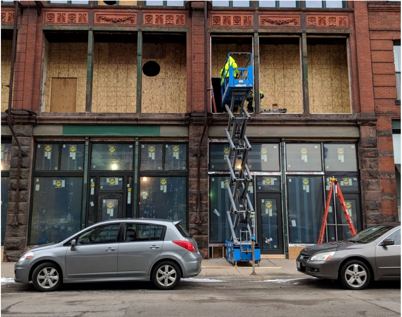
Figure 34: Storefront being renovated, Historic Baker Importing Company Building at 212 North Second Street, Minneapolis. Photo by Catherine Sandlund
