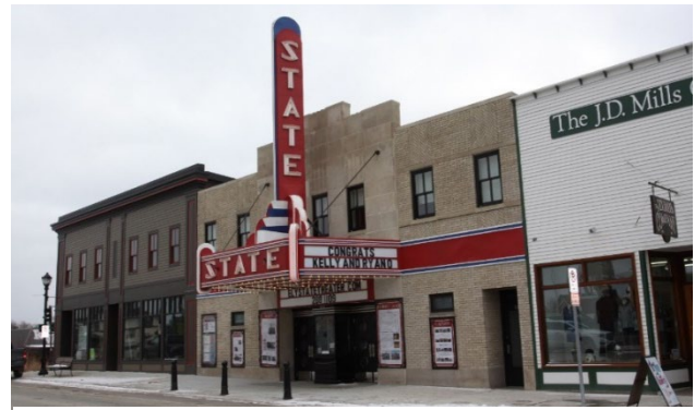
Figure 18: Ely's State Theater was rehabilitated using state and federal preservation tax credits. Photos by Charlene Roise
