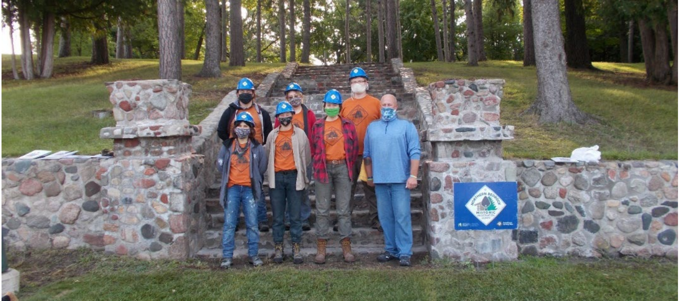
Figure 29: Northern Bedrock Historic Preservation Corps, with assistance from Ray Stenglein of Environmental Associates Inc., repaired the masonry stairs at Riverside Park, St. Cloud. Photo by Ann Marie Johnson
