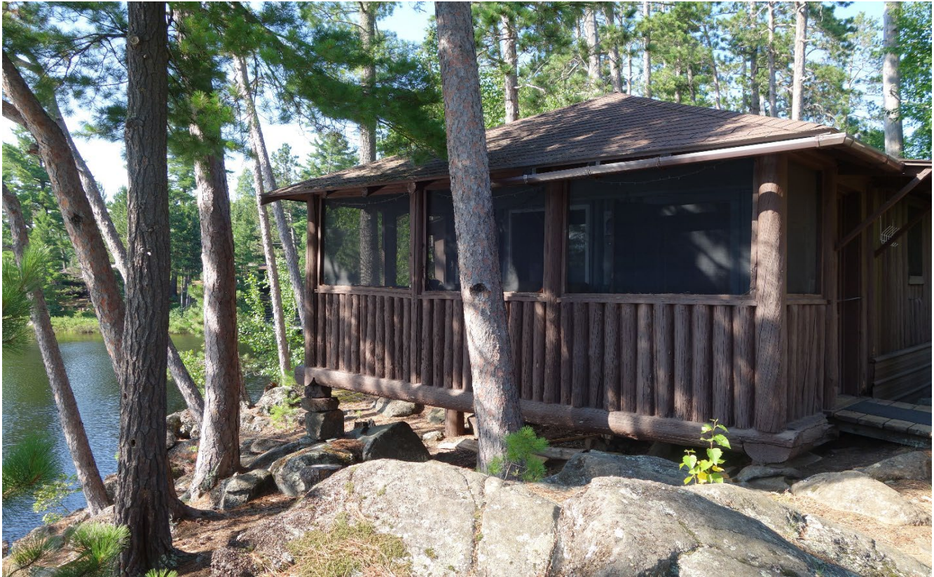
Figure 13: Kawishiwi Lodge, Cabin 15, near Ely. Photo by Rolf T. Anderson
