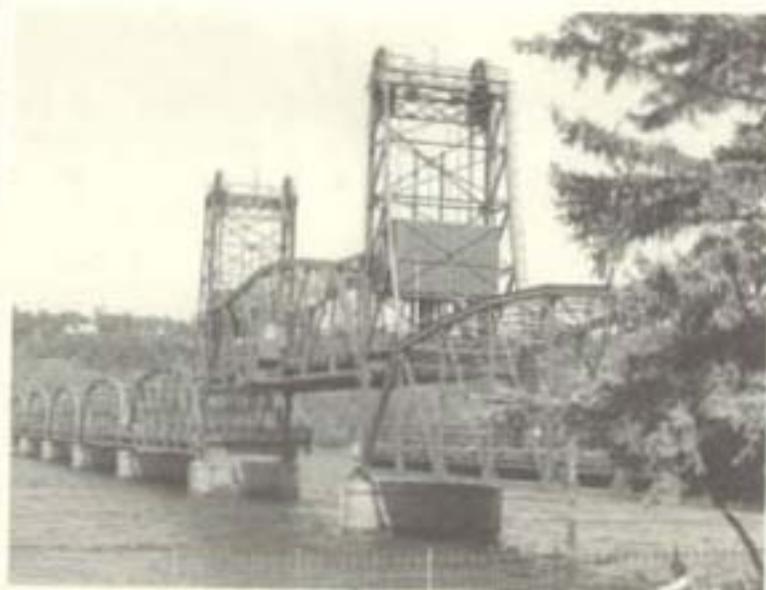
Sallwater Bridge, Sallwater, Washington County
