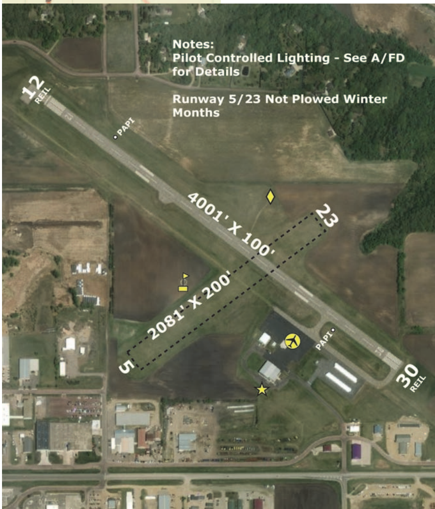
Redwood Falls Municipal Airport
