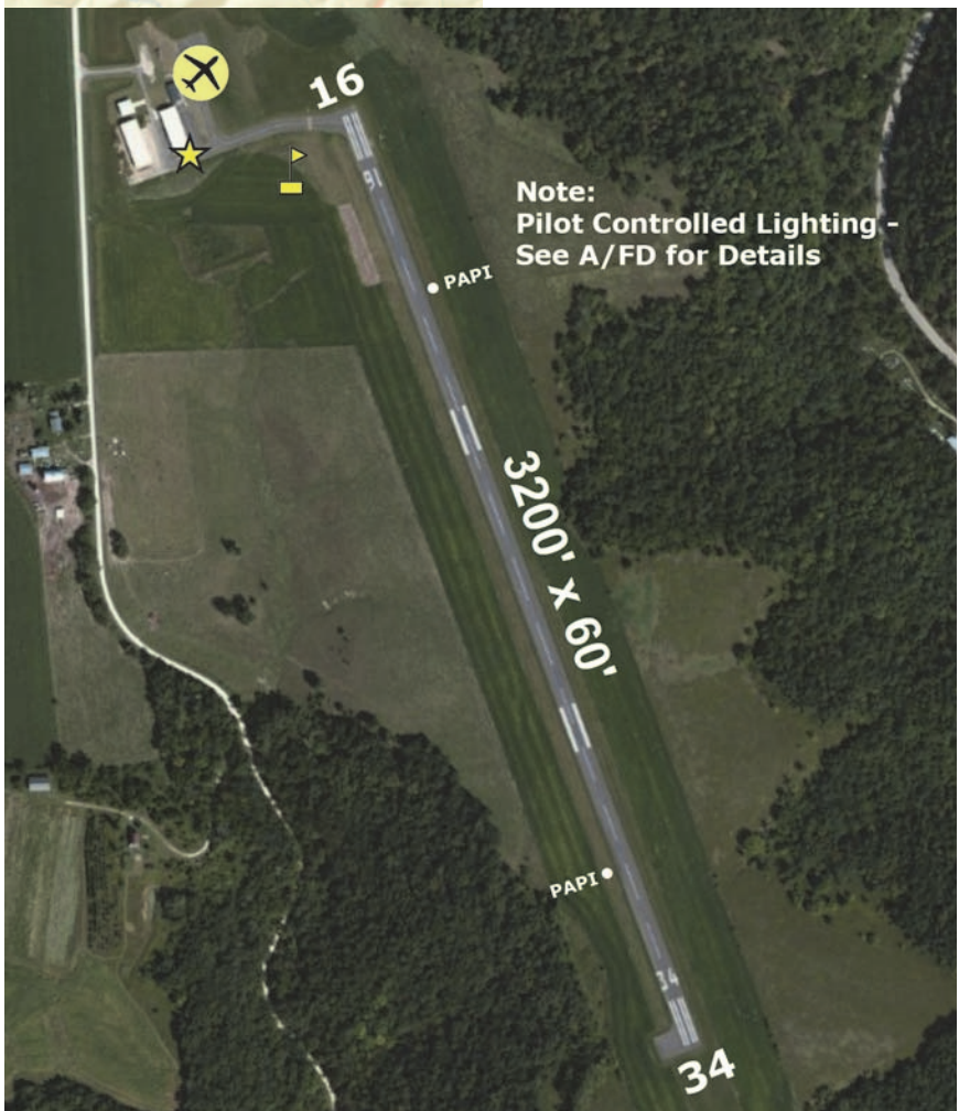
Rushford Municipal Airport - Robert W. Bunke Field
