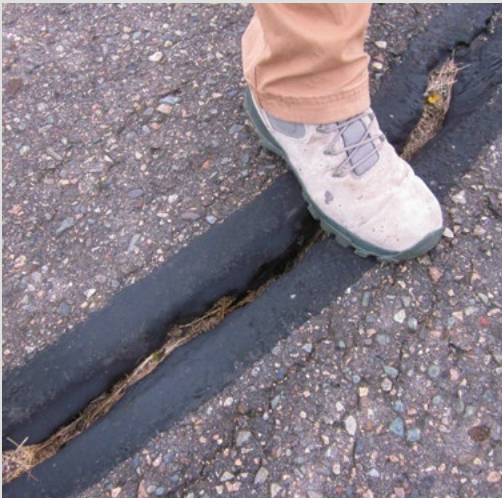
This deep crack at the Hibbing air tanker base ramp is unsafe for taxiing aircraft.
