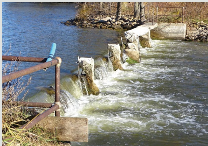
High Island Lake dam failure.
