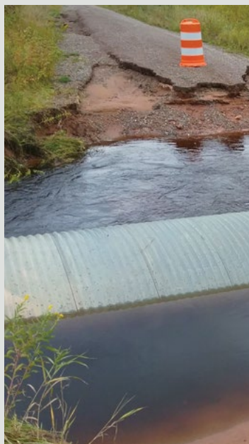
Harlis Forestry road washout damage.
