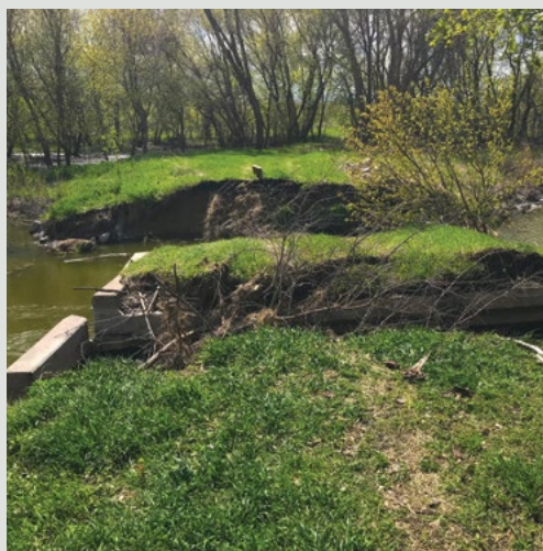
Perkins Lake water control structure failure.
