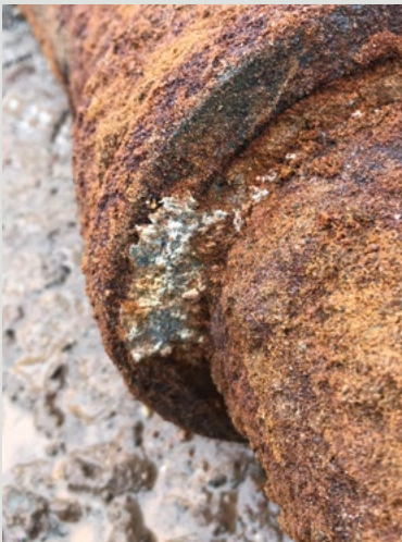
Septic piping poor condition prior to repair.
