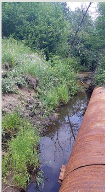
Trails culvert washout.
