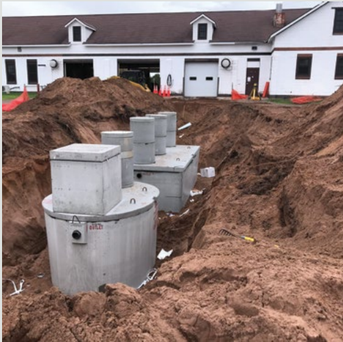
Septic replacement under construction.
