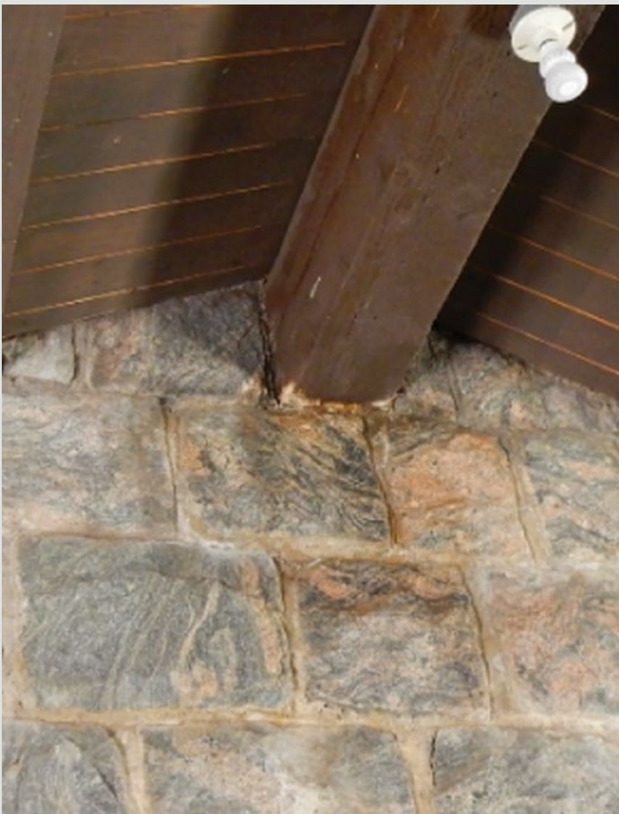
Fort Ridgely State Park day-use area shelter ceiling wood beam rot.
