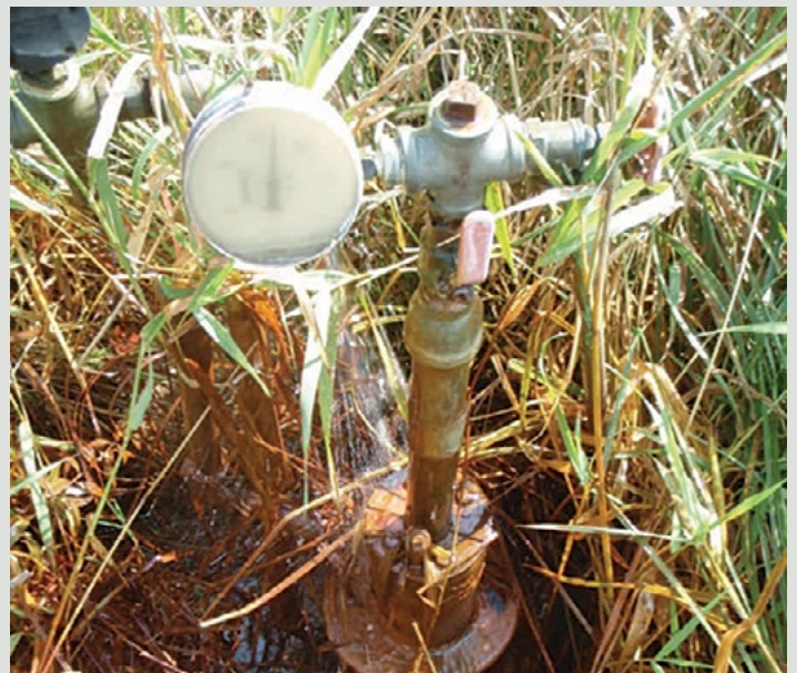
Monitoring well in need of replacement.
