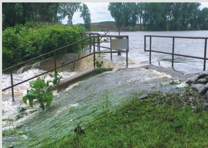
Warren Lake dam failure.
