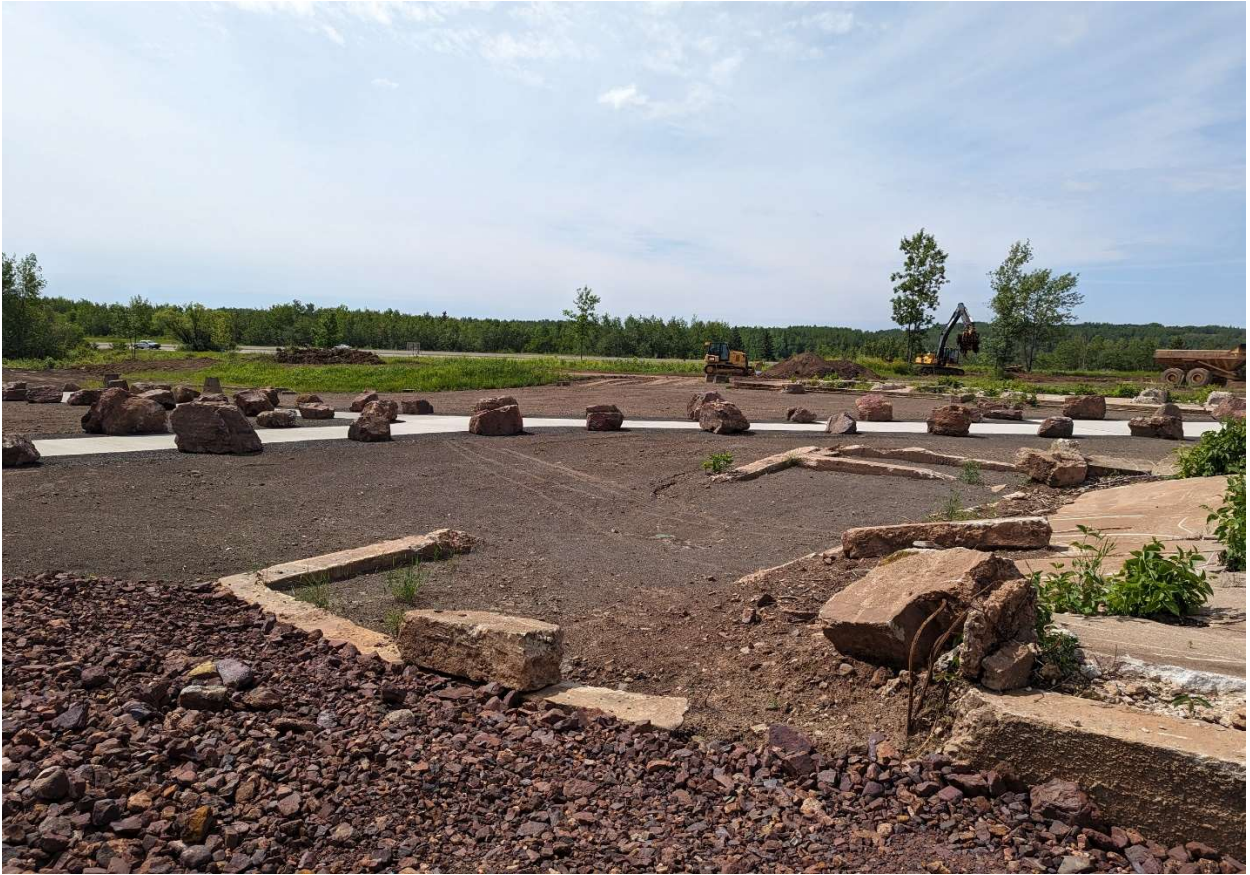
Landscaping; During Construction
