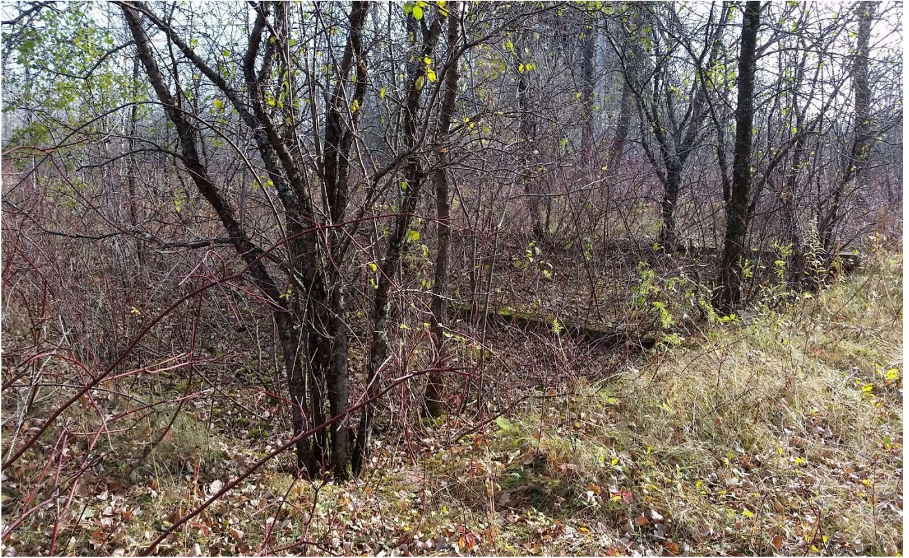
Before: Concrete foundations
