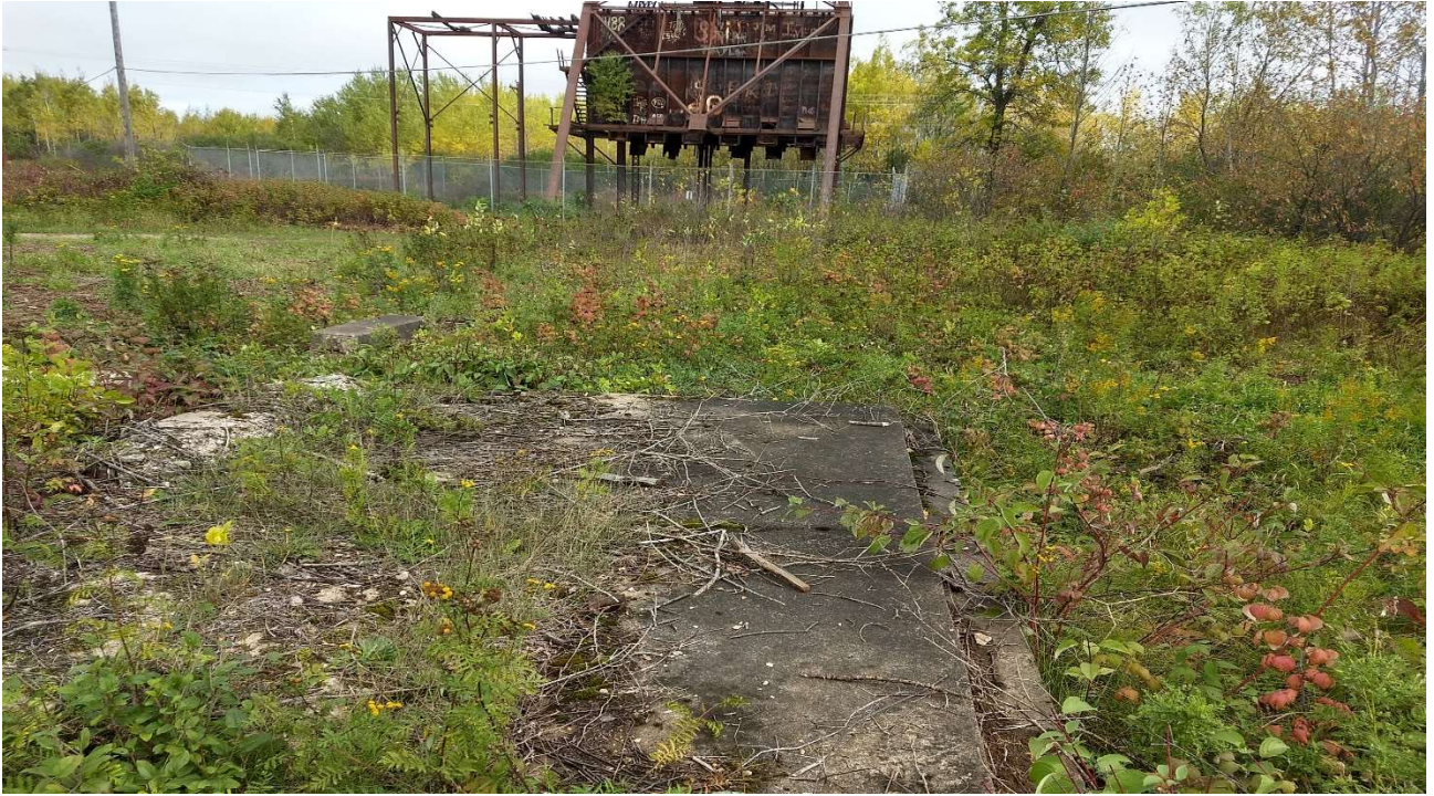
Before: Clearing foundations
