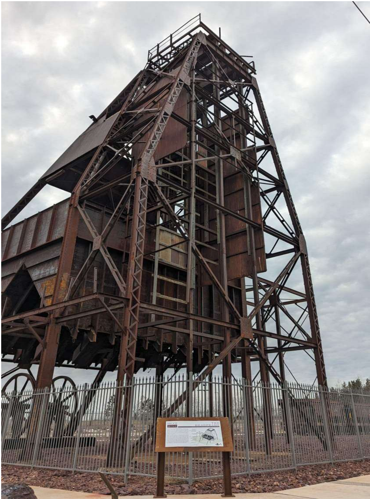
Headframe with Sheave Wheels, Plaque, Railcars, Taconite Rock Base
