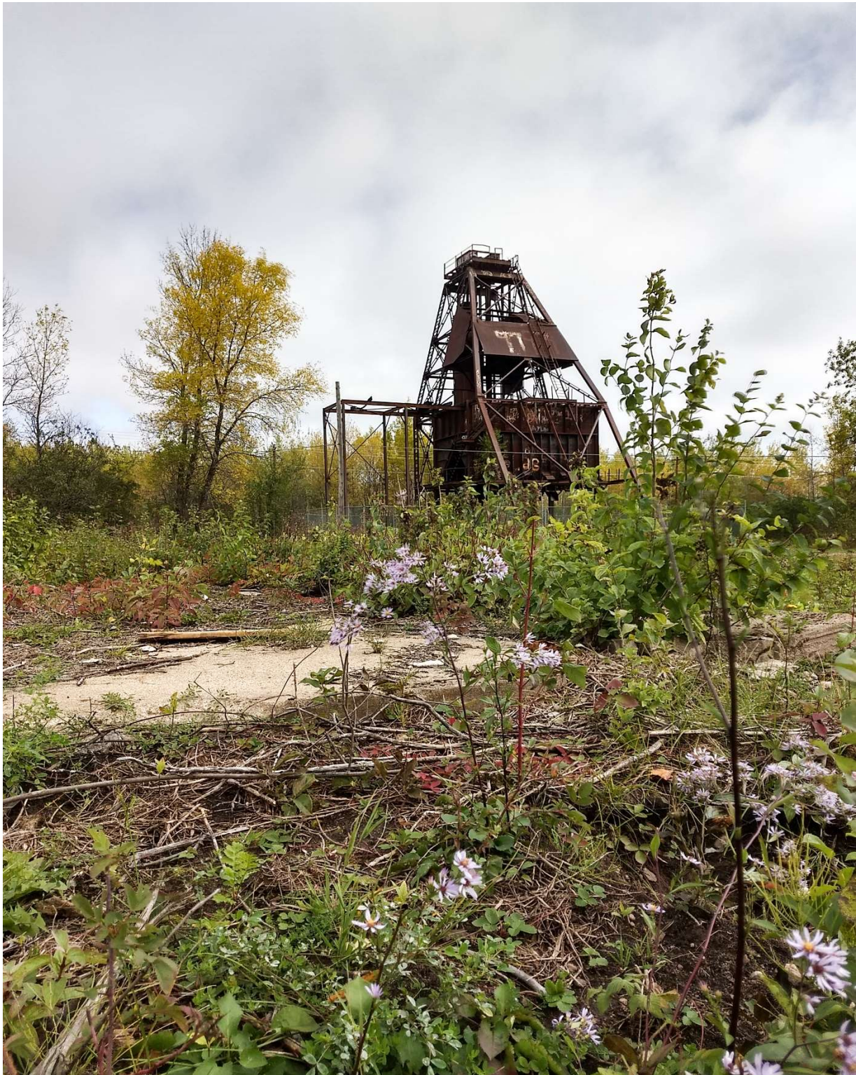
Before: Headframe and building concrete foundation
