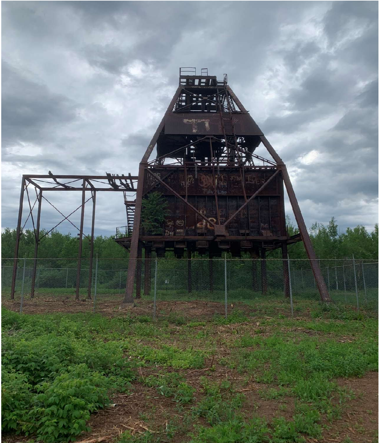
Headframe: During clearing
