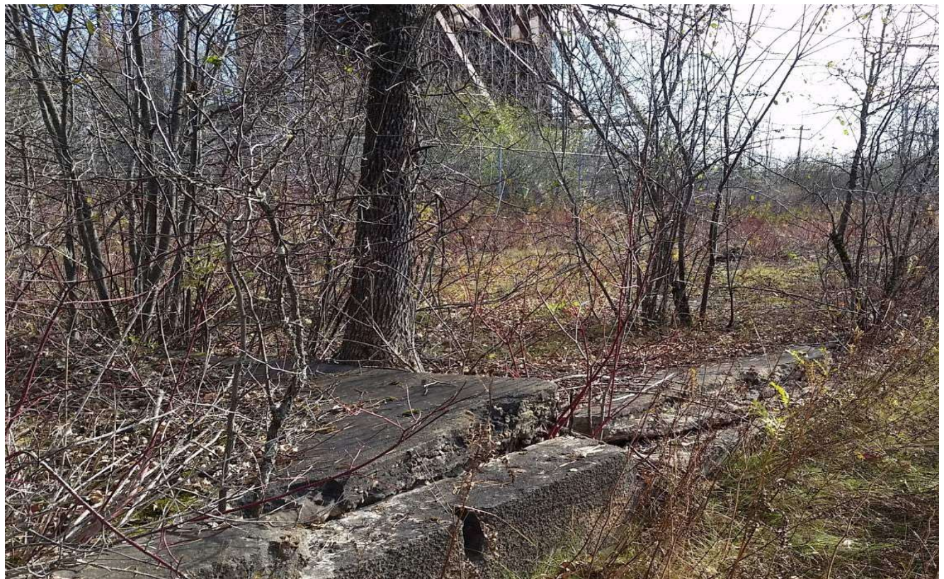
Before: Historic concrete foundations
