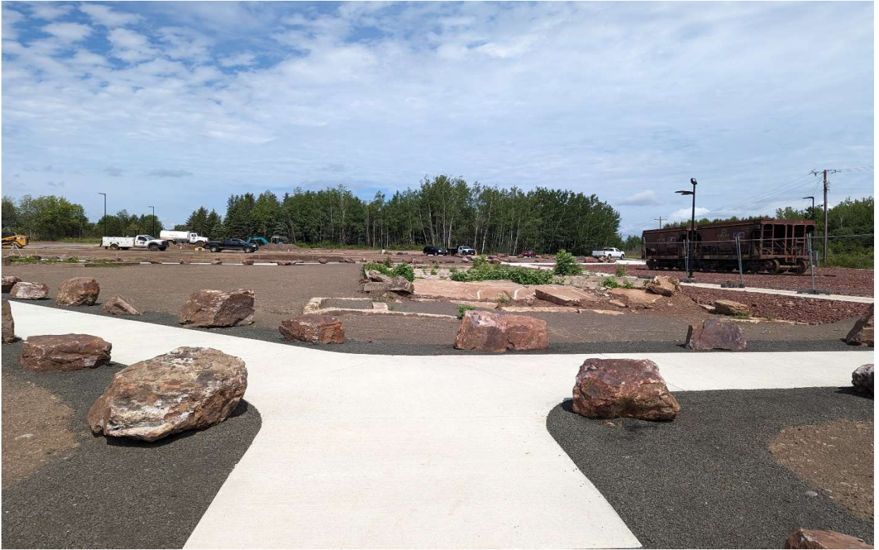
Foundations and Concrete Walkway: During Construction
