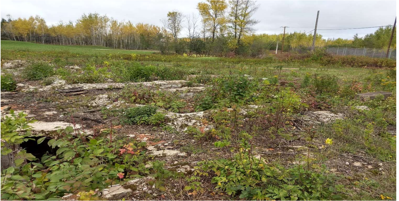
Before: Clearing foundations
