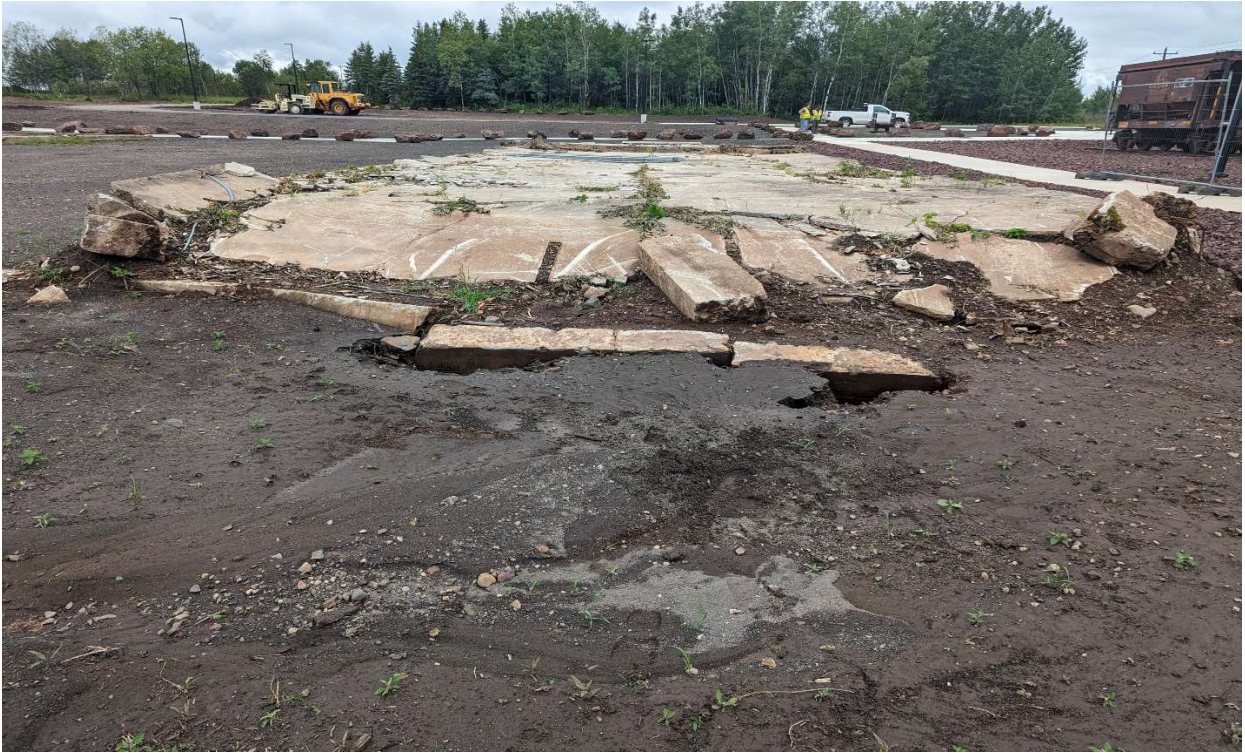
Foundations: During Construction
