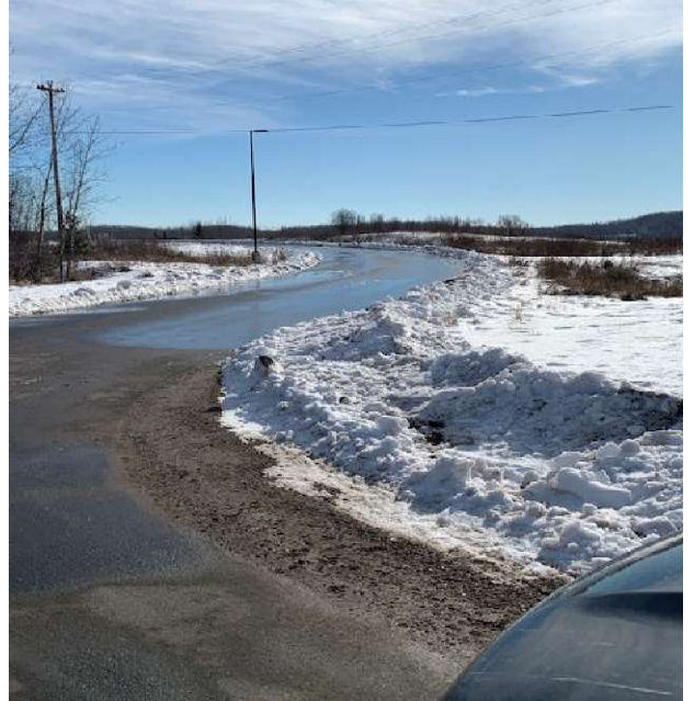
Paved Entrance Road
