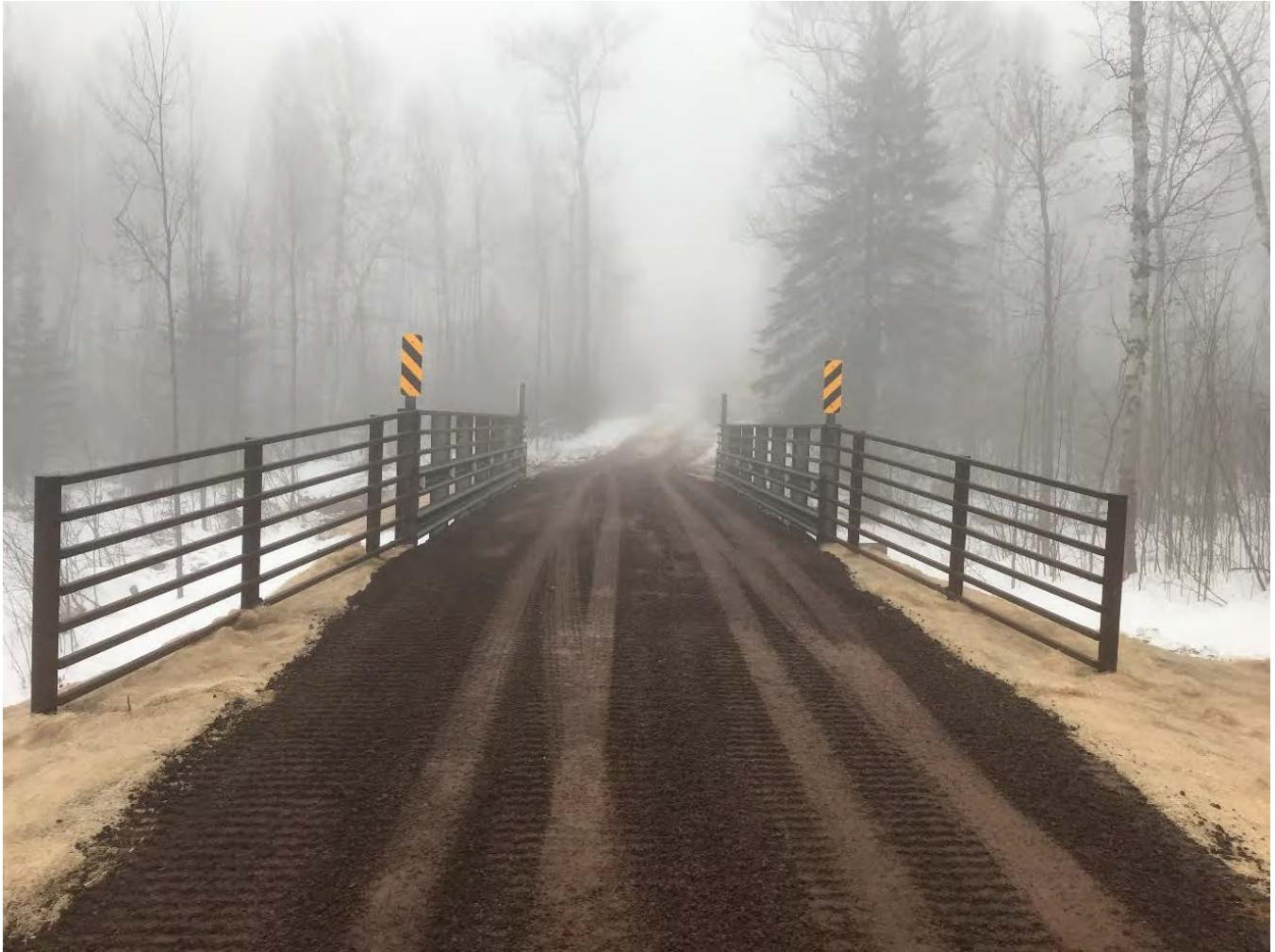
CJ Ramstad/Northshore State Trail: Big 39 Creek River Bridge / Replacement (Complete)
