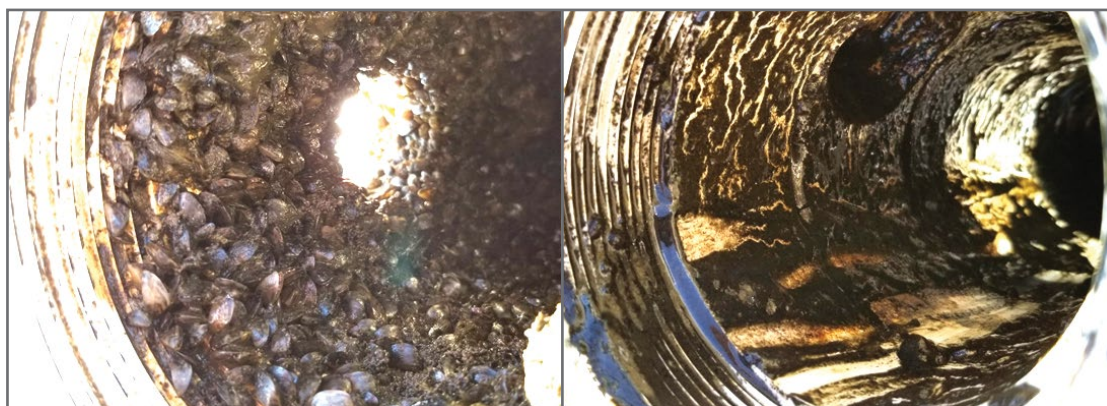
Intake line from control (left) and CO 2 treatment (right)
