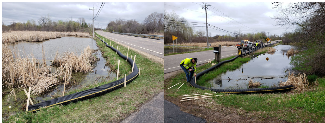
Figure 4. Construction of new 8-inch pipe barrier in Dakota County to keep turtles and other small wildlife off roadways.
