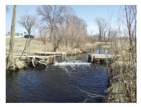
**Figure 9.** Bubble curtain. Upstream view of bubble curtain tested in Zielinski and Sorensen, (2015) in Kohlman Creek, Minnesota (45°01'36" N 93°02'48" W). Upstream of the bubble curtain is a wetland used by carp for spawning; a chain of lakes is downstream. The bubble curtain blocked up to 60% of juvenile common carp moving downstream.
