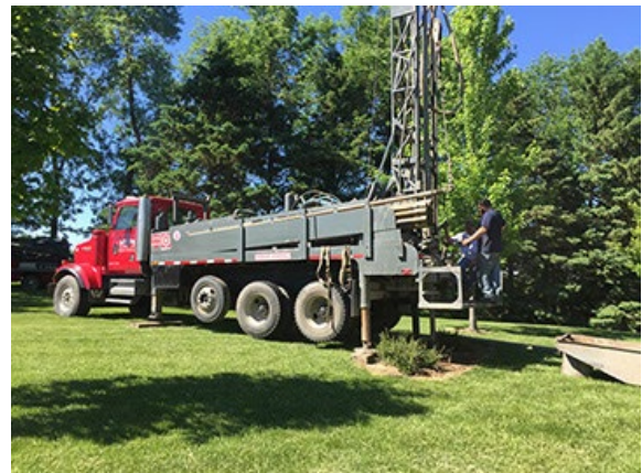
Figure 29. Typical well drilling installation.
