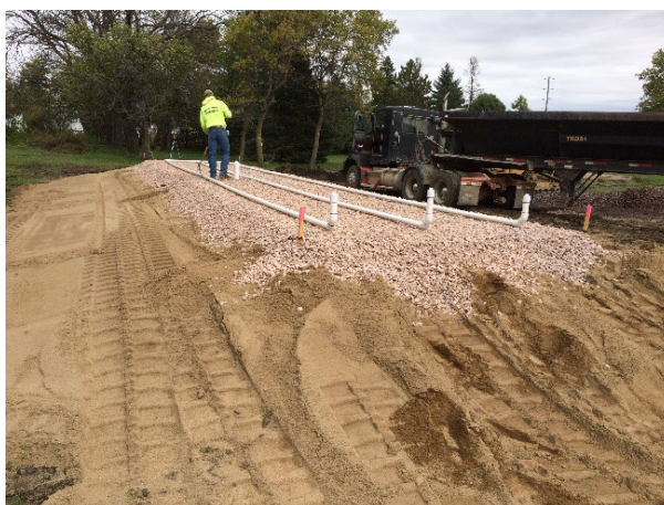
Figure 25. Installation of a typical septic tank and mound drain field, Watonwan County.
