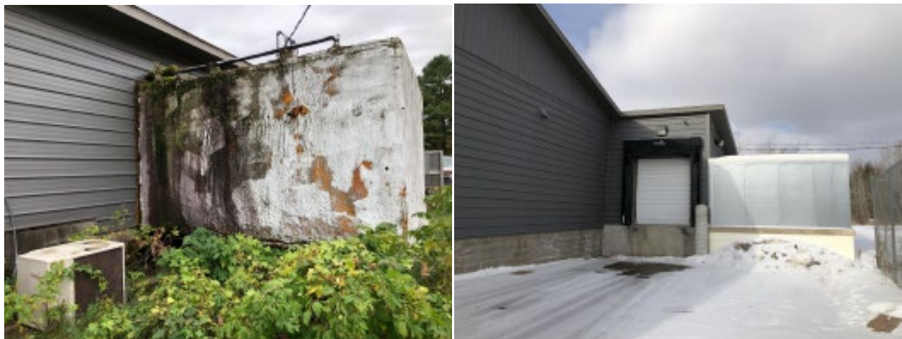
Photo 3 and 4. Mark's Market, a FY20 recipient located in Hackensack, purchased, and installed a new cooler (right) to replace the old, failing cooler (left). This upgrade allows for Mark's Market to store more produce and better meet the needs of their customers. Photos courtesy of Mark's Market.
