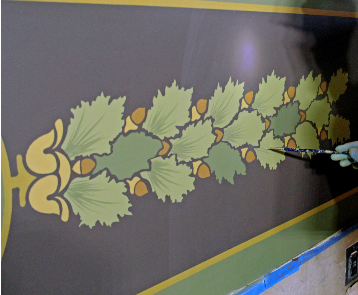
Decorative paint was touched up where needed in 2021.
