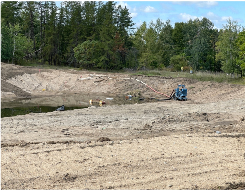
During Construction: Oil containment plug
