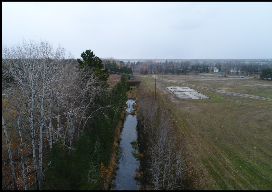
Before Construction: Ditch by lake Irving
