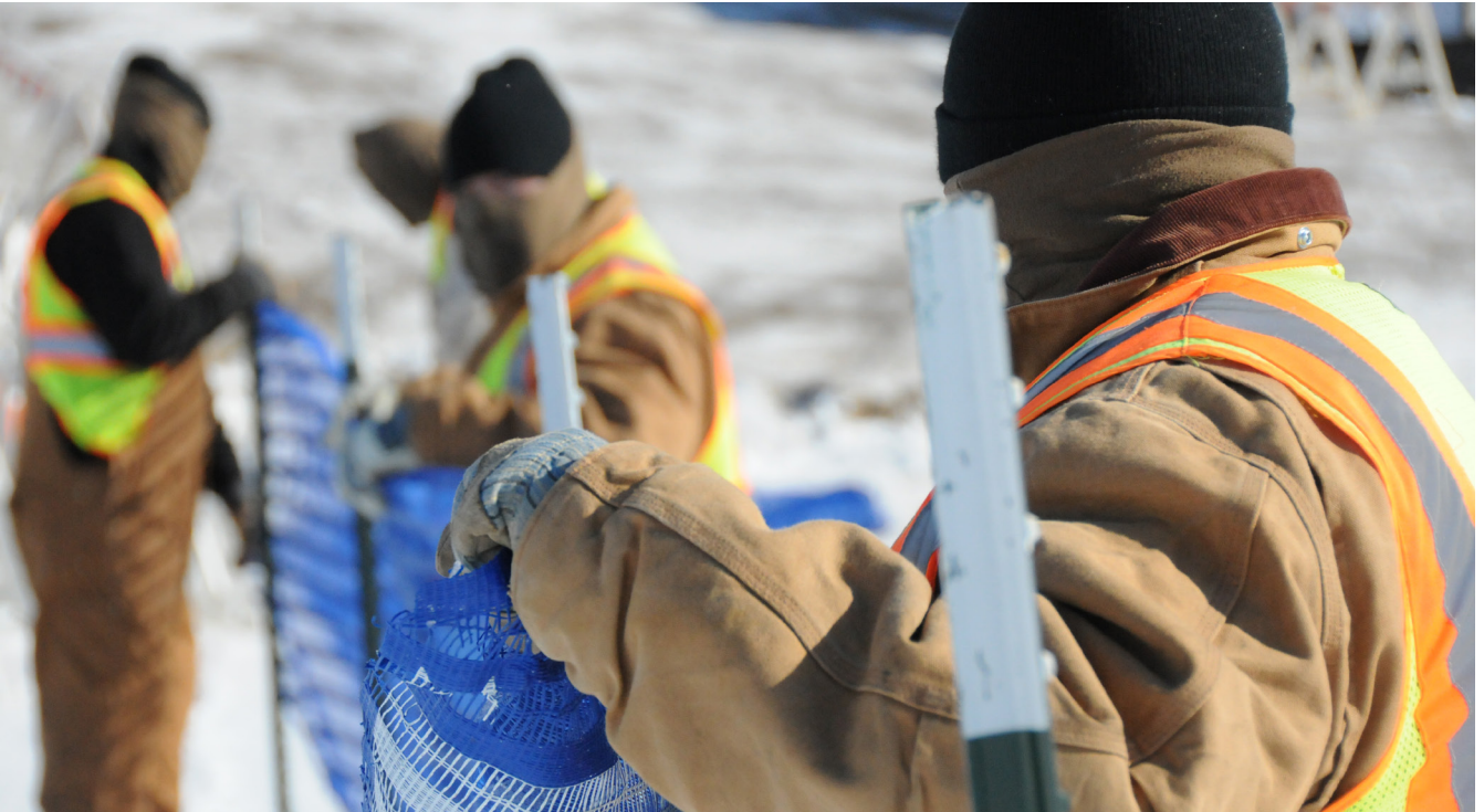
An incarcerated person work crew installs a snow fence in the community
