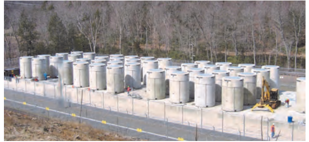
Loaded spent fuel storage casks are in place on storage pad at the Haddam Neck Plant in Meriden, CT. (Courtesy: Connecticut Yankee)
