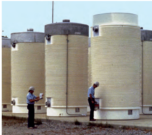
Inspectors examine dry storage casks containing spent nuclear fuel.
