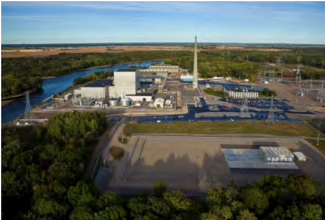
Figure 1. Monticello Nuclear Generating Plant and ISFSI 4
