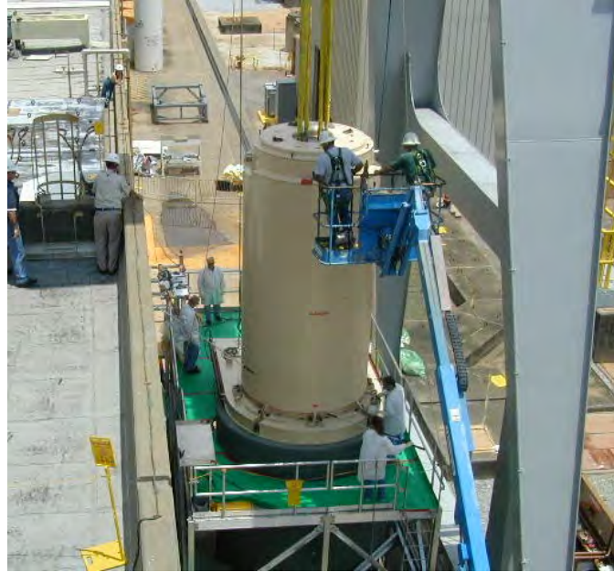
Figure C-11: Placement of Transfer Cask on Overpack with Mating Device
