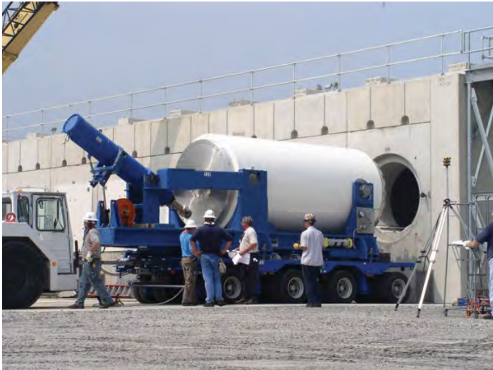
Figure 8. Canister Being Placed in Horizontal Concrete Storage Module
